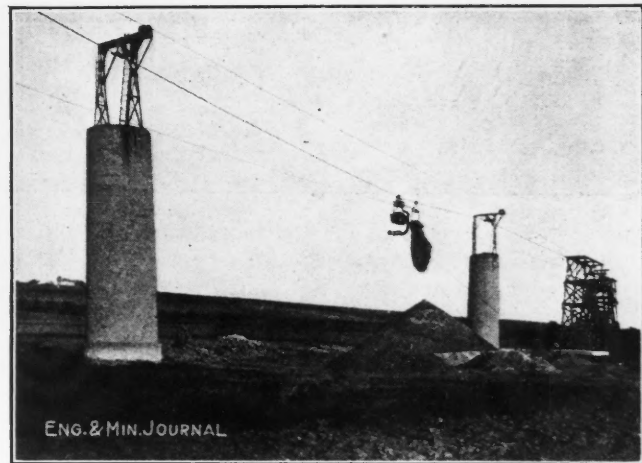
FIG. 1. CONCRETE ROPEWAY SUPPORTS WITH STEEL SUPERSTRUCTURE
