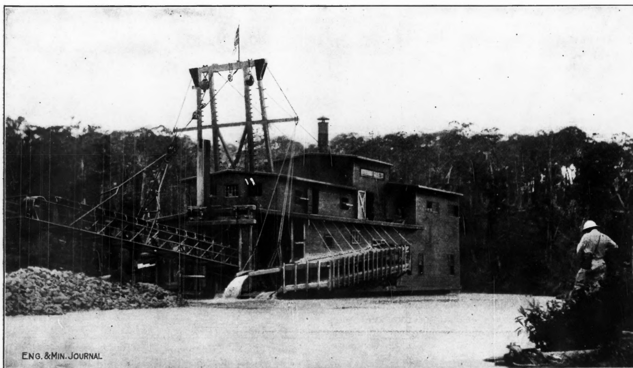
THE 6-CU.FT. DREDGE OF THE GUMAOS PLACER CO. RETURNED 25C. PER CU.YD. FROM ITS 1913 OPERATION IN THE PARACALE DISTRICT, ISLAND OF LUZON
