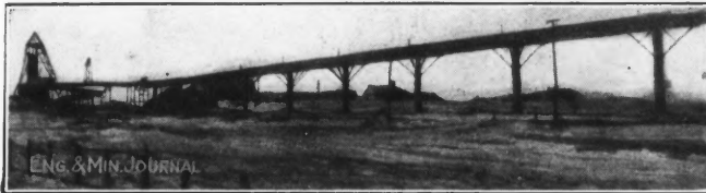
FIG. 9. ONE HALF OF THE NEGAUNEE TRESTLE. NOTE THE FEW COLUMNS REQUIRED FOR THE GREAT LENGTH OF TRESTLE
