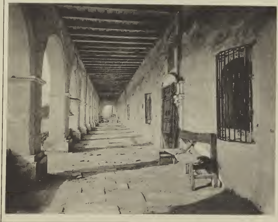
SAN FERNANDO REY DE ESPAGNA - CORRIDORS OF MONASTERY
