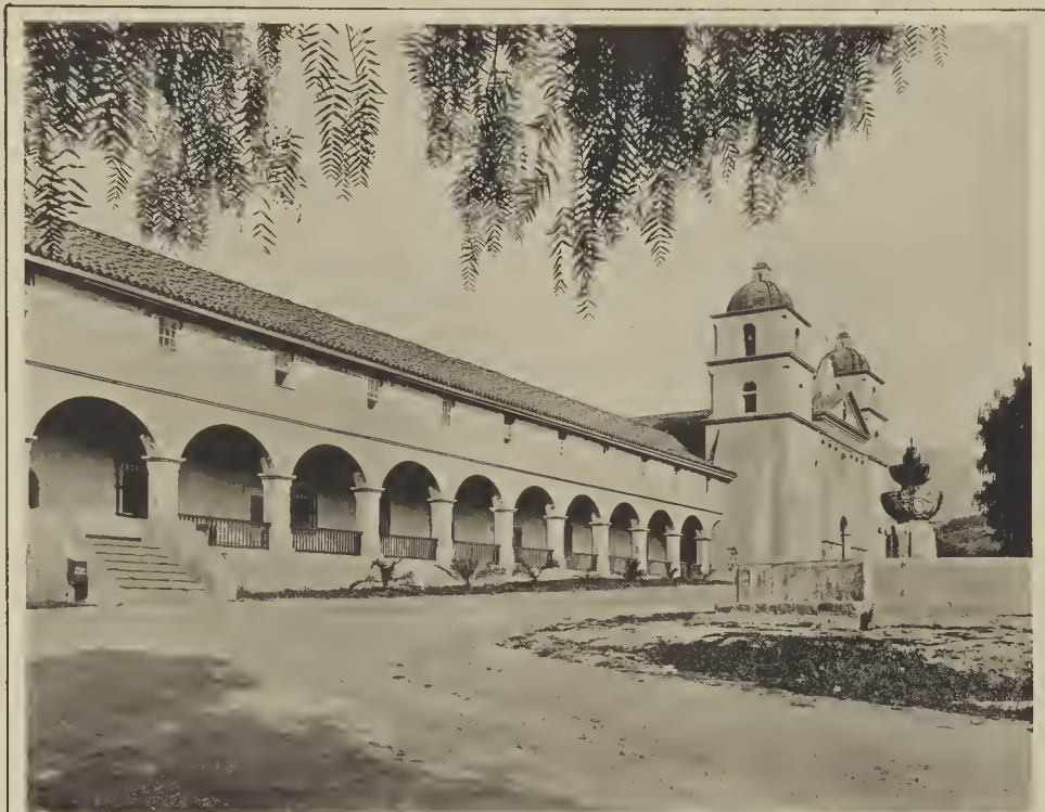
SANTA BARBARA MISSION - FACADE
