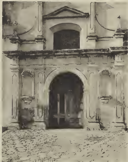
SAN CARLOS DE MONTEREY DETAIL OF FACADE
