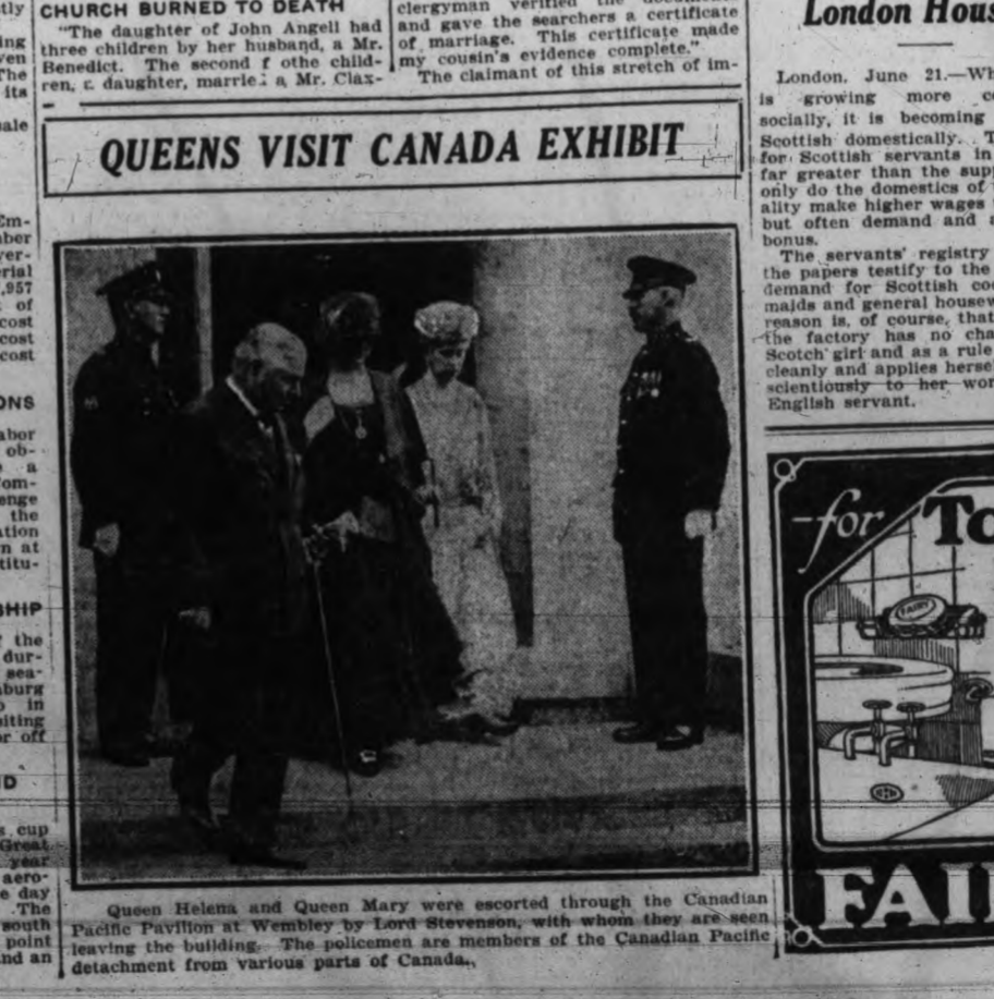
Queen Helena and Queen Mary were escorted through the Canadian Pacific Pavilion at Wembley by Lord Stevenson, with whom they are seen leaving the building. The policemen are members of the Canadian Pacific detachment from various parts of Canada.
