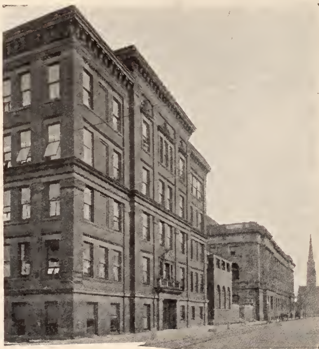
MARQUETTE HOSPITAL AND DISPENSARY, MILWAUKEE.
