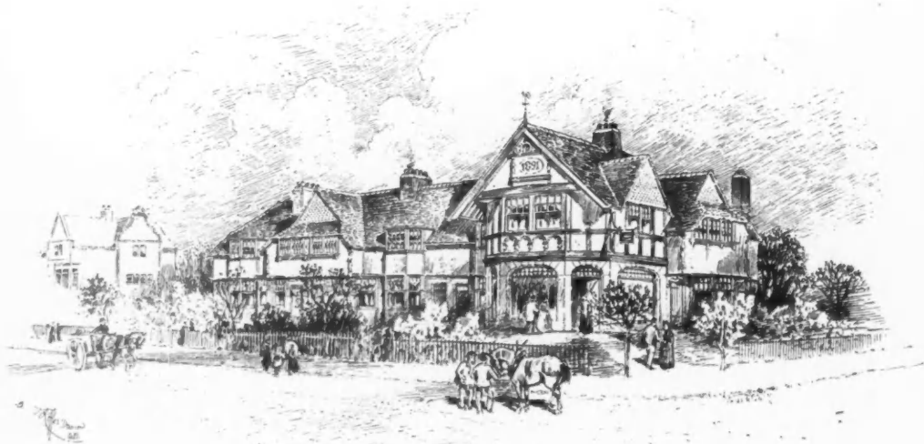
Dining Hall and Workmen's Cottages, Port Sunlight, for Messrs. Lever Bros., Ltd., WILLIAM OWEN, F.R.I.B.A., Architect.
