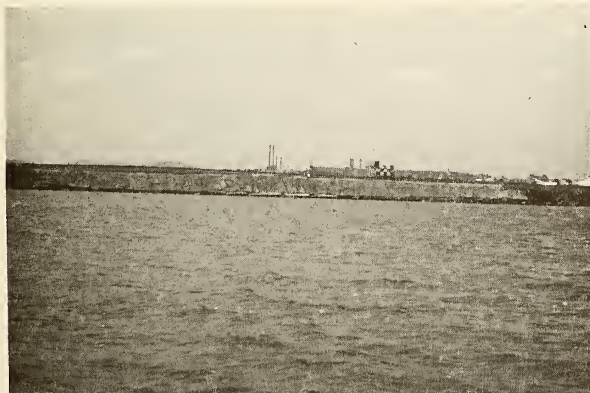
2. VIEW OF AIRPORT PERIMETER END OF RUNWAY 22L
