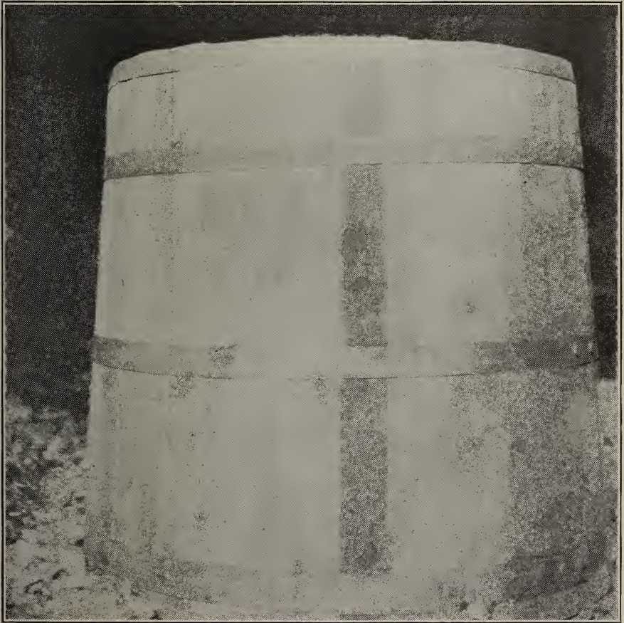
Fig. 22.—Finished oil tank.
