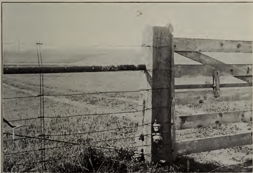
Fig. 31. CHESTNUT POST ATTACKED BY BROWN ROT ( POLYPORUS SULPHUREUS ).
