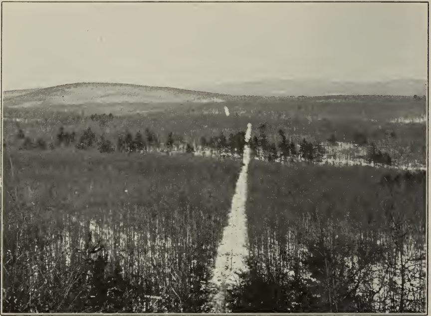
Fig. 27. OIL PIPE LINE AS A FIRE AND SUBDIVISION LINE. A base from which to fight fires. An excellent subdivision line.
