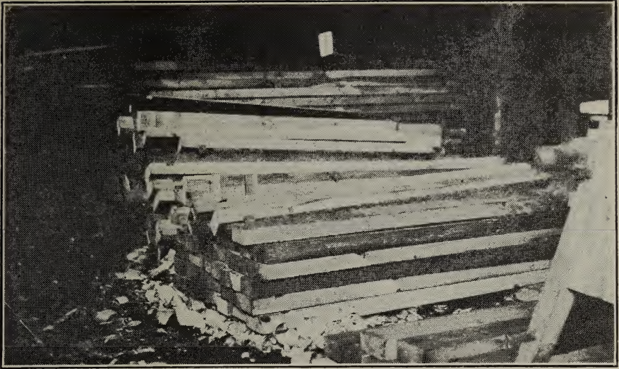
Fig. 21.—Oil tank staves preparatory to assembling.
