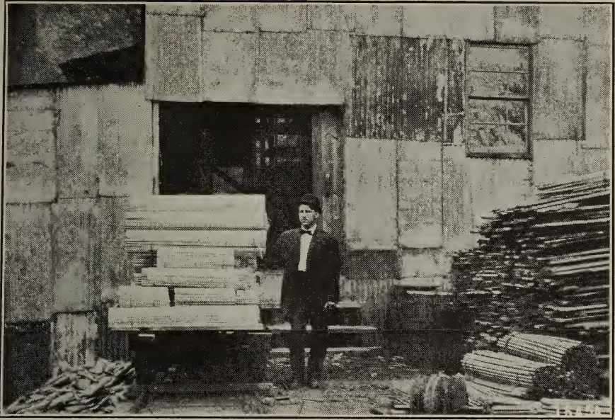
Fig. 5.—Utilization of mill waste. Rough squares are bolted from slabs and edgings, and turned into chair stock.
