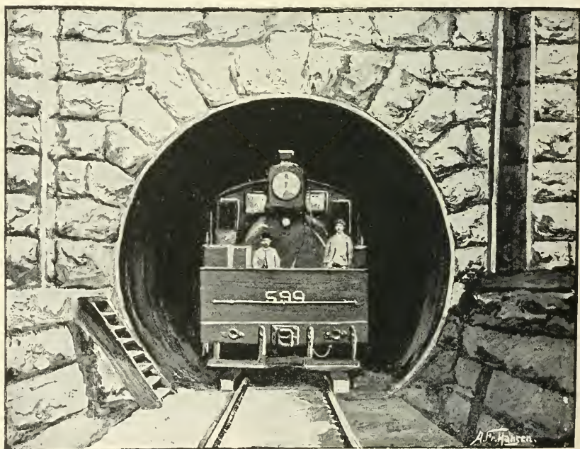
TUNNEL ENGINE EMERGING FROM PORTAL.
