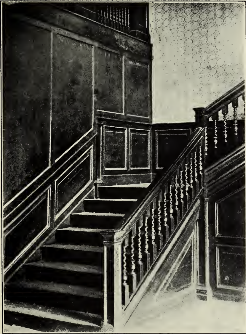
STAIRCASE, GROUND FLOOR.
