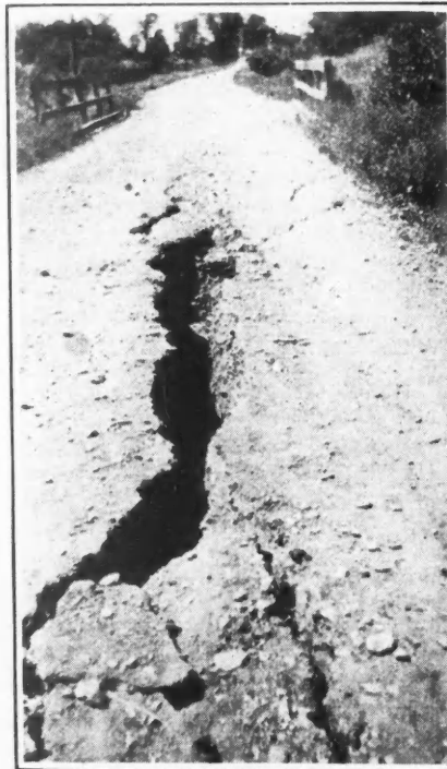
Crevice formed by earthquake, June 28, 1925, Logan, Mont. Average width of opening 9 inches
