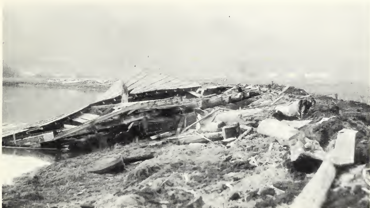
Photo 28.--The remains of a destroyed building, logs, and other debris have been deposited on this dike. They will have to be removed, Siuslaw River, Oregon, 1951. SCS photo NO. 7-367-10
