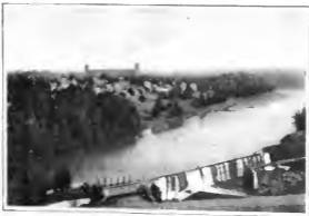
.1 View of the new Utopia in South Carolina
