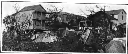
A Group of wrecked Buildings in Port Antonio, Jamaica
