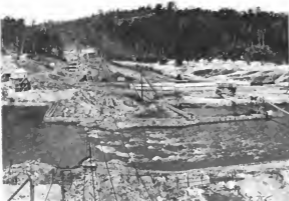
Constructing a Power Dam on Bull Sluice Shoals, Alabama
