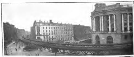
Dovey Square, Boston, showing the South Union Station—The largest Railroad Terminal in the World
