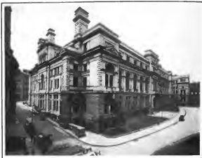
The new Court House, Boston
