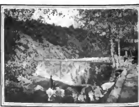
A Placer County Irrigating Dam
