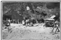
The Tunnel of a Quicksilver Mine
