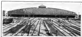
Rear of the South Union Terminal, Boston, showing the twenty-eight Tracks entering the Station
