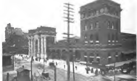
The North Union Station, Boston
