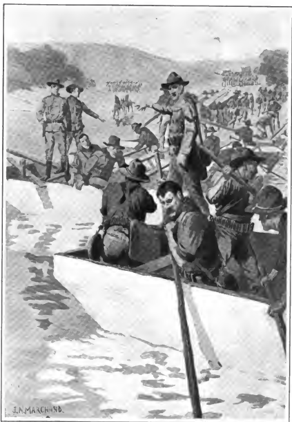
Engineer Corps.—Building a Pontoon Bridge
