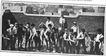
"Hurling the Hoops" on the Roof of an East-Side School-house Many of the East-Side schools in New York now have playgrounds on their roofs, which the children use for their games and sports. An East-Side baseball nine plays its road team on one of these rooftop playgrounds.
