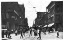
Whitehall Street, Atlanta—Looking South
