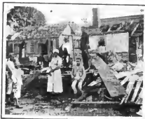
In the Negro Colony at Kingston after the Hurricane
