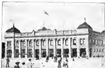
Winstock Lakin and Co.'s Building, Sacramento
