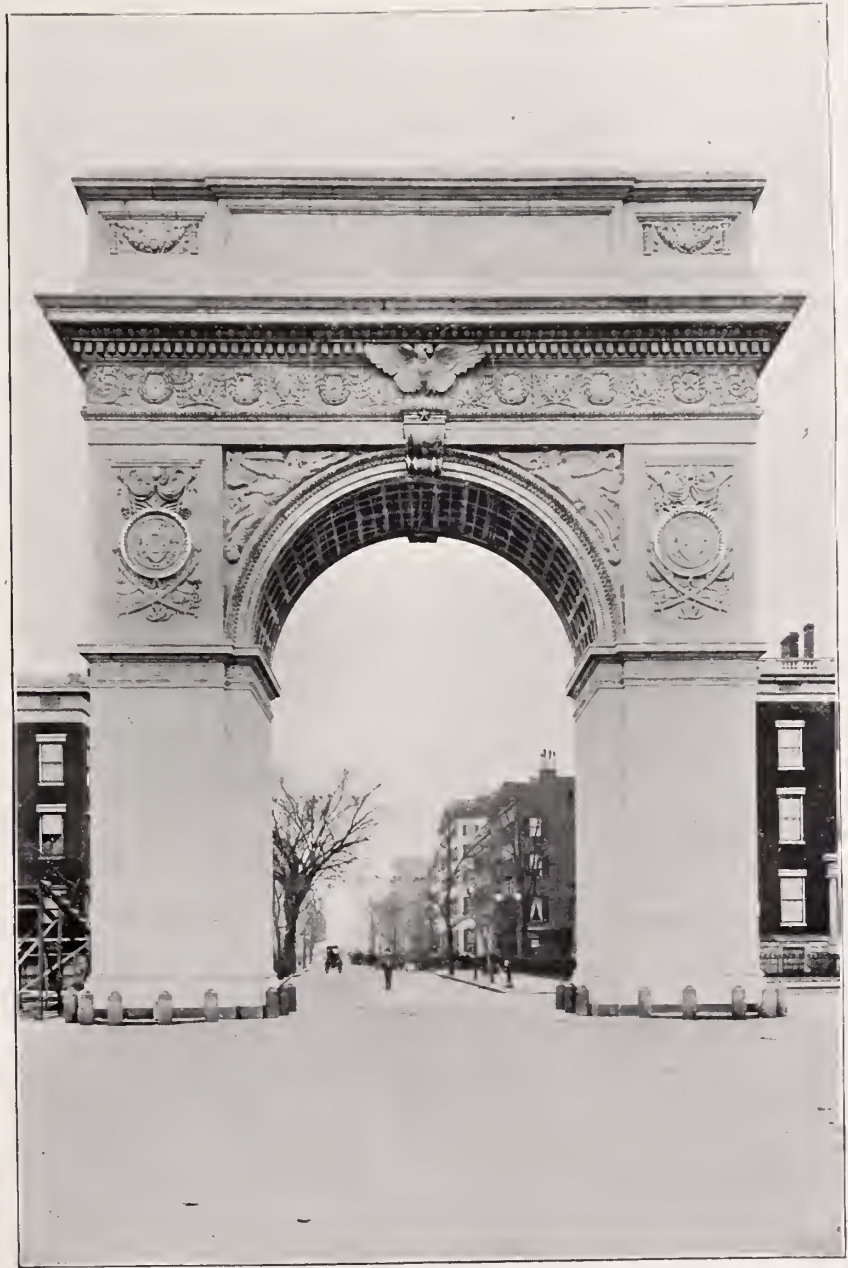
WASHINGTON ARCH, (SOUTH VIEW.)
