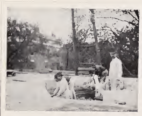
THE EASTERLY PIER RISING FROM THE PLATFORM.
