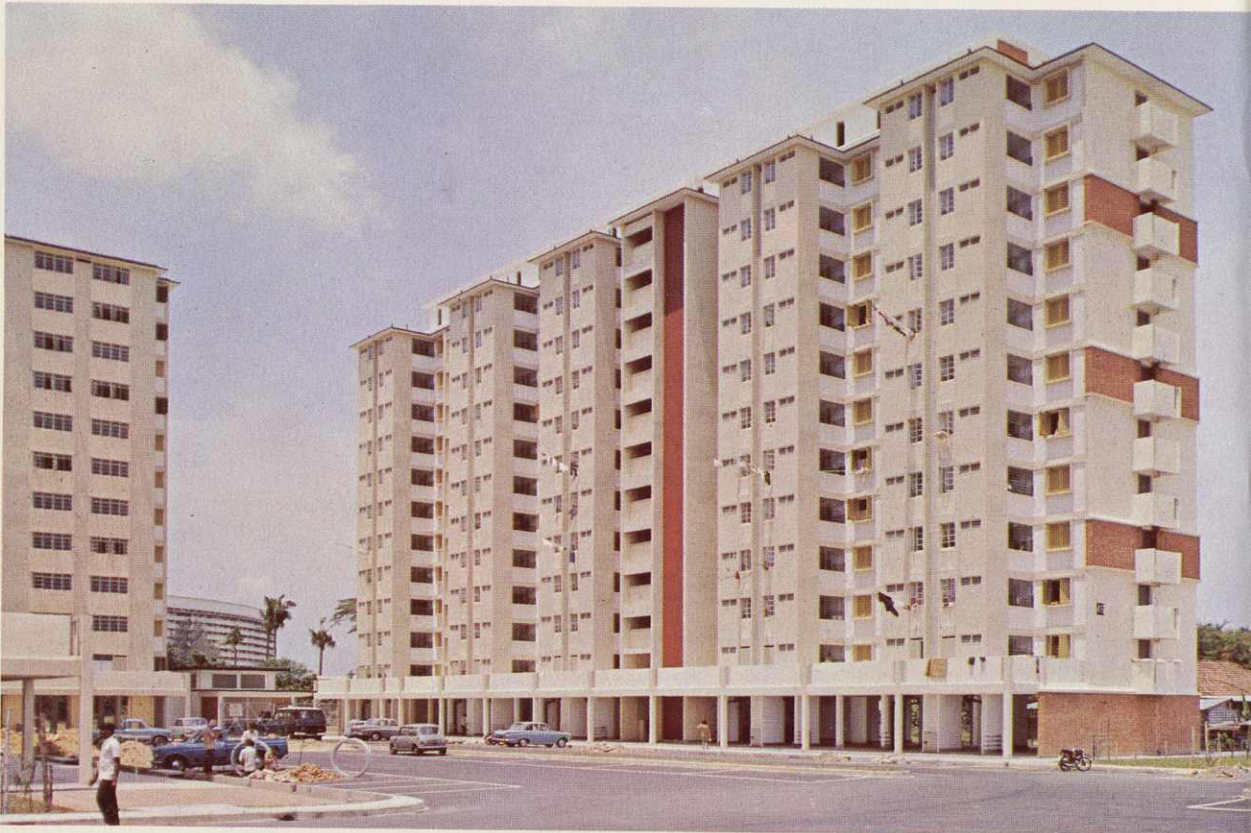
A block of newly designed 1-room (Improved) flats in Kallang Basin, Neighbourhood II. The void ground floor serves as a covered play area for children.
