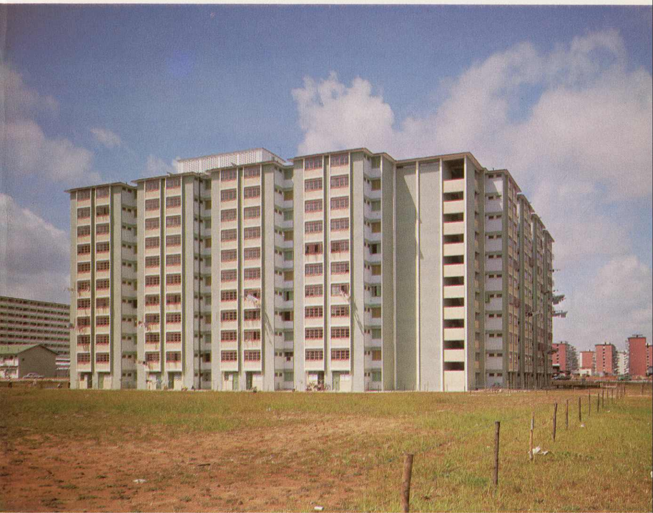
Focus is now on the back elevation of the L-shaped block of 3-room flats in Toa Payoh, Neighbourhood I.
