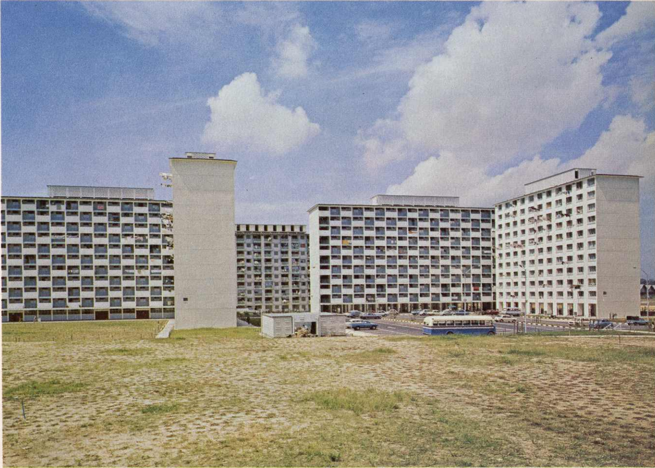
Highrise flats in Toa Payoh, Neighbourhood IV. In the foreground is a large expanse of newly turfed area and a spacious carpark.
