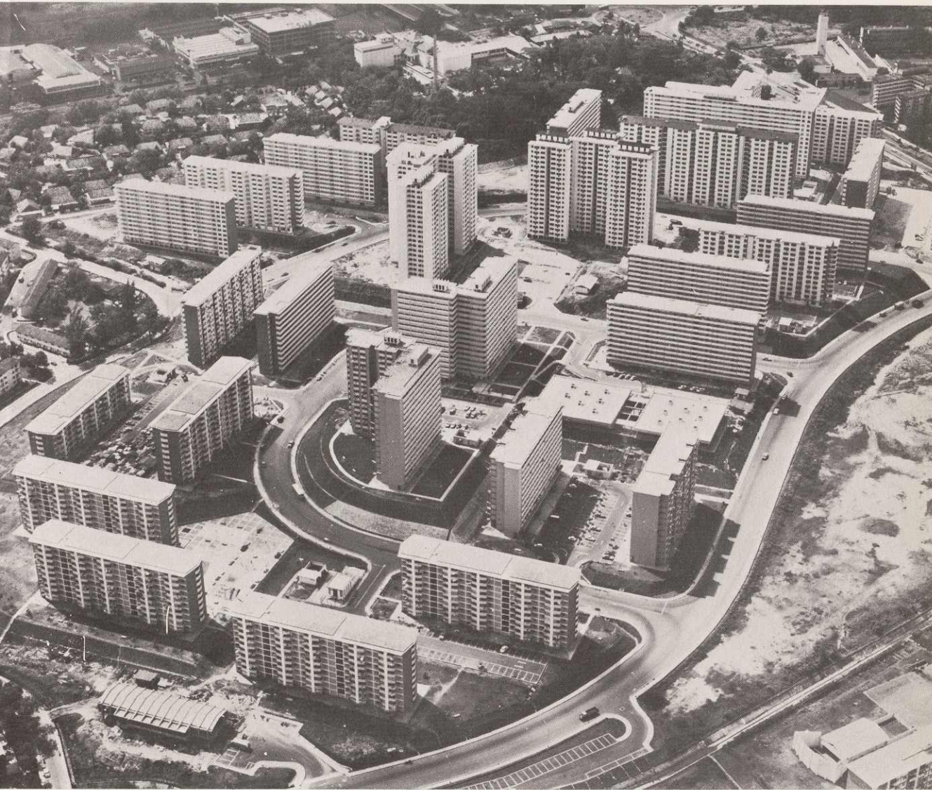
An aerial view of Queenstown, Neighbourhood VI.
