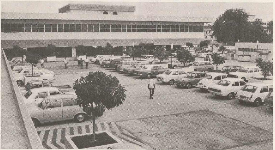
A view of the spacious carpark at the National Development Building. In the background is the Annexe Block which houses the Resettlement Department and the Applications and Lettings, and Sales Offices of the Estates Department.
