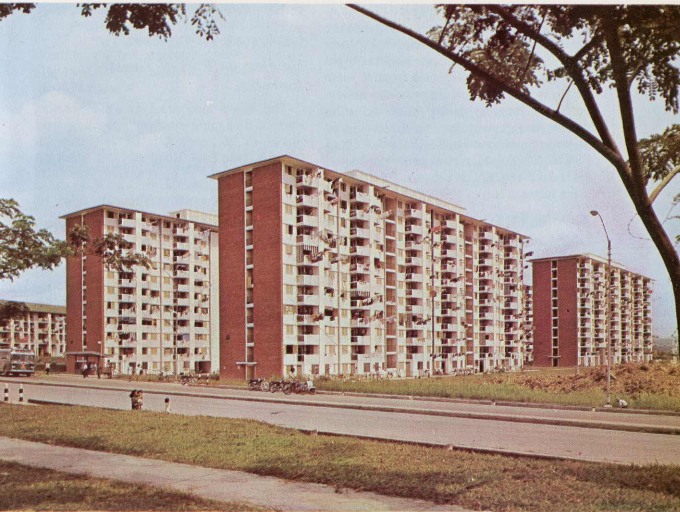
Blocks of 1-Room (Improved) flats built by the Board on behalf of the Jurong Town Corporation in the Jurong Industrial Town.
