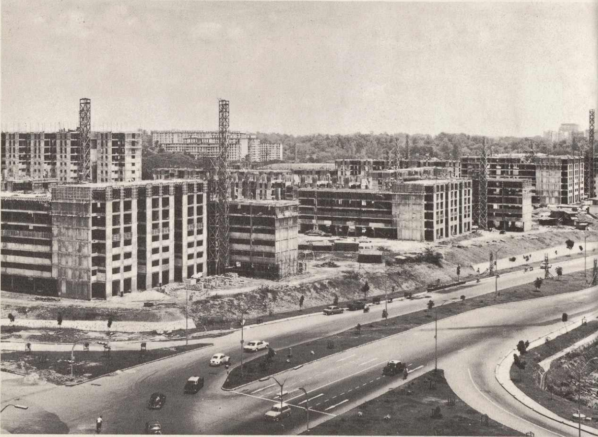
Flats under construction in Toa Payoh.
