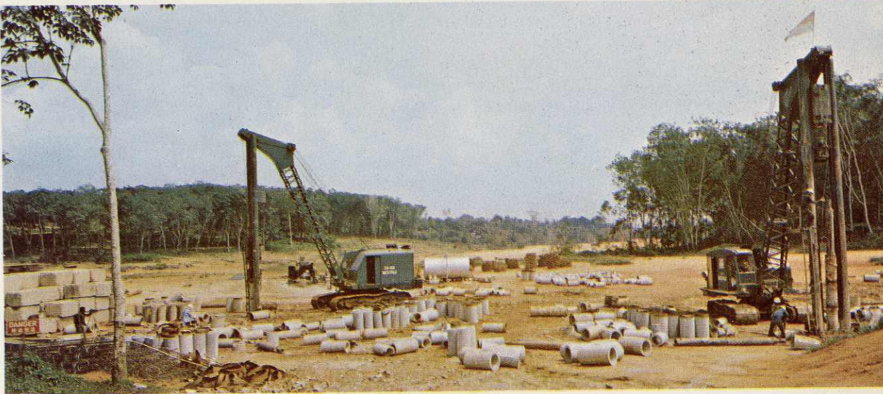
Commencement of piling work in the development of Woodlands New Town.
