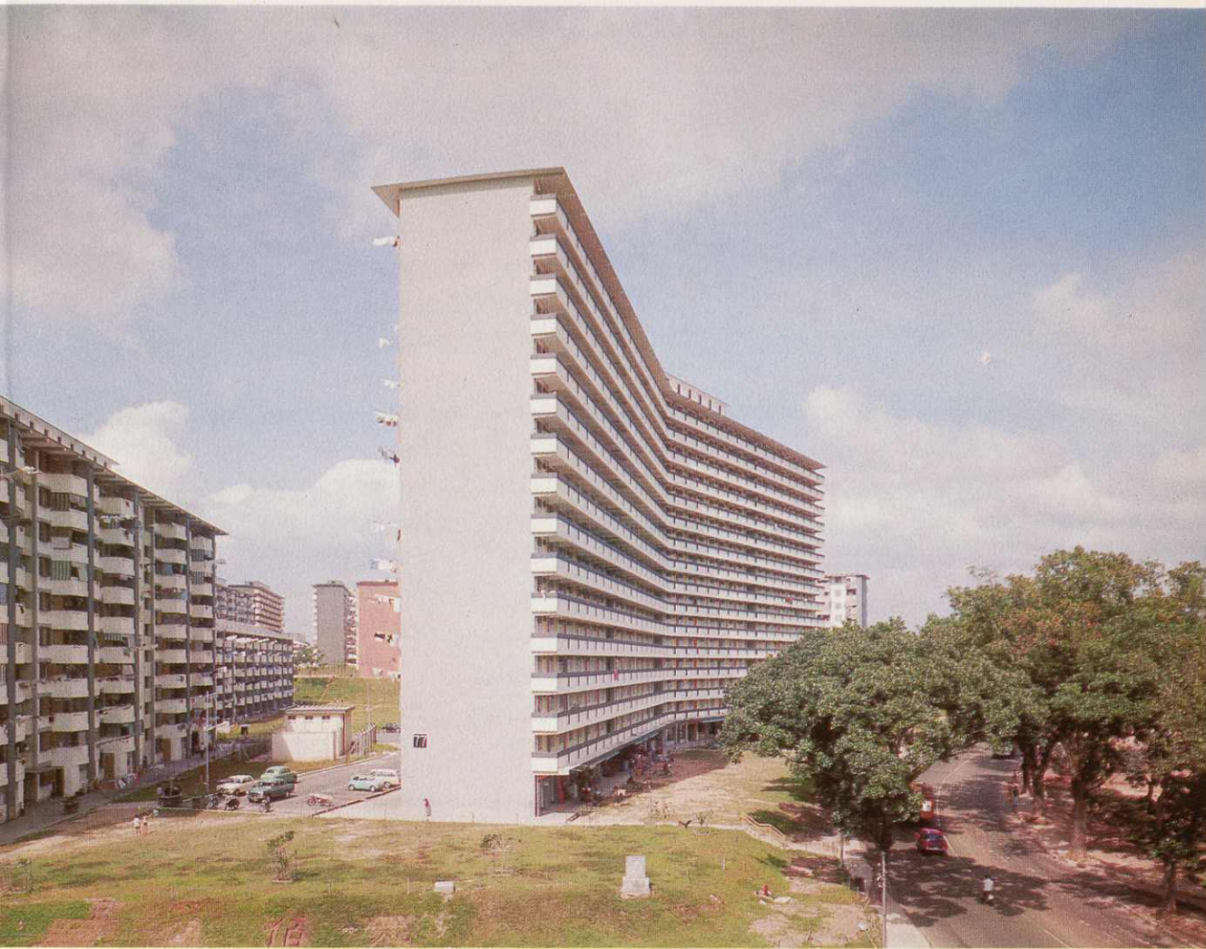
Part of the redevelopment of Bukit Merah— this is a 16-storey block of 3-room and 2-room Improved flats.
