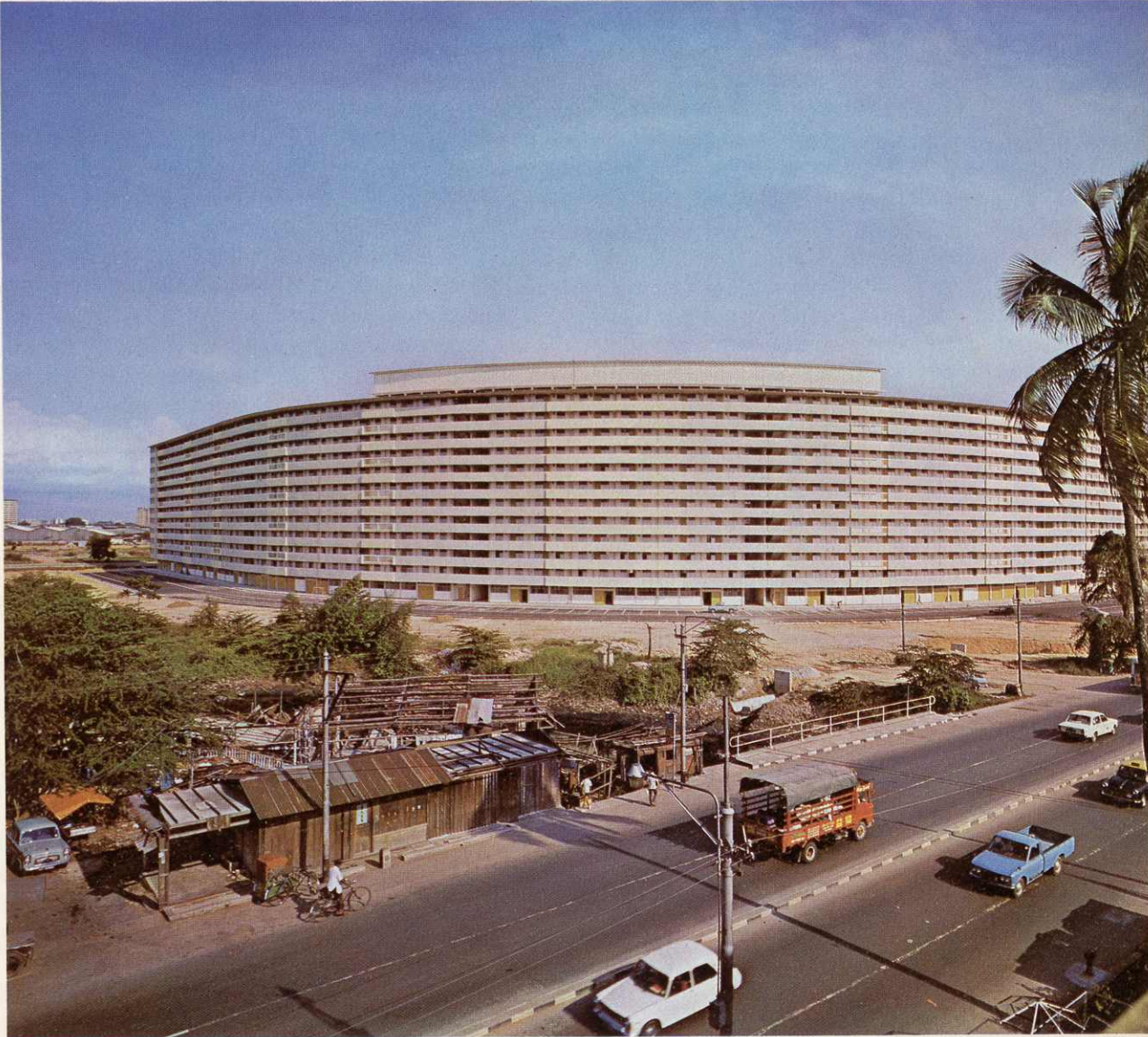
An elongated curved building in Kallang Basin, Neighbourhood I. In the foreground are dilapidated huts which will be demolished to make way for public housing.
