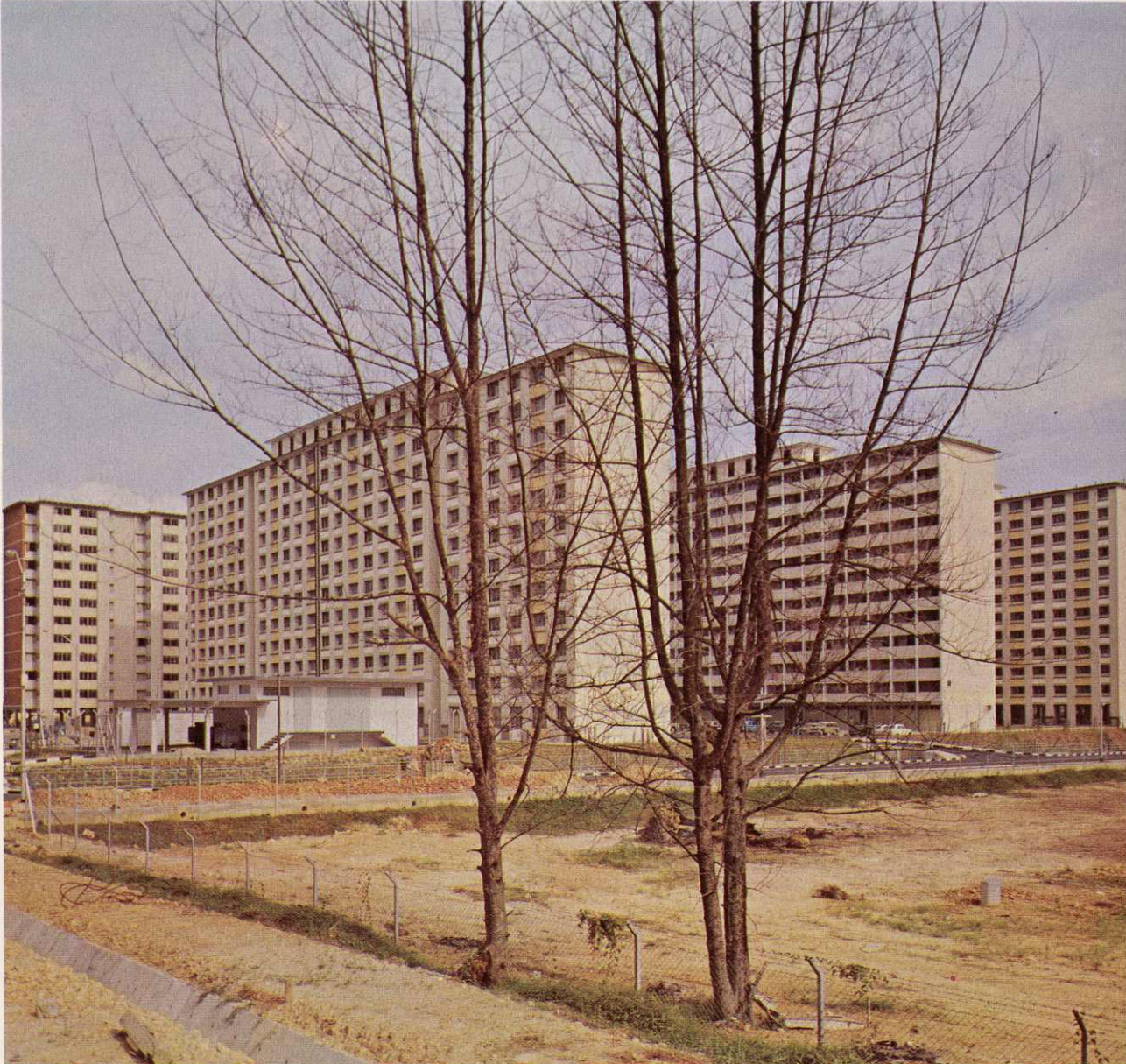
Highrise flats in Toa Payoh adjacent to a large expanse of open area.
