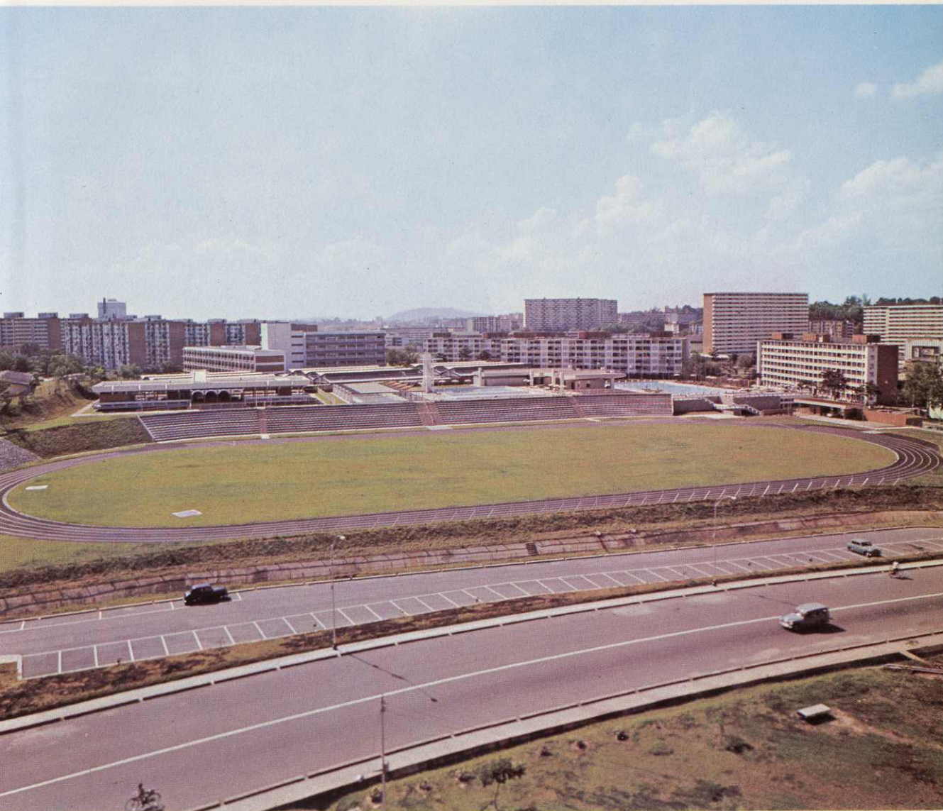
A general view of the Sports Complex in Queenstown. The provision of a sports complex will become a standard feature in all new towns and large housing estates.
