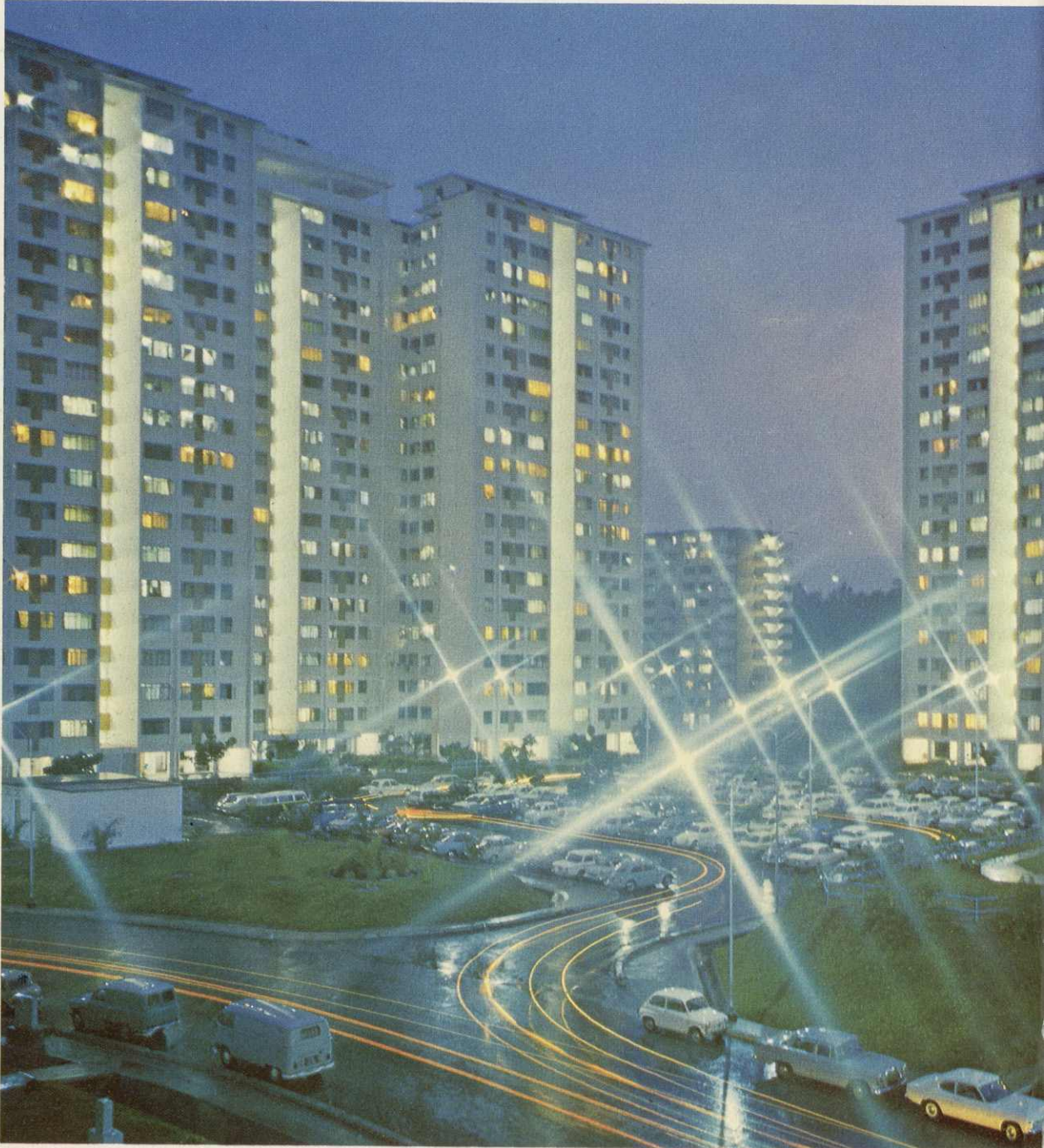
Queenstown Neighbourhood VI by night
