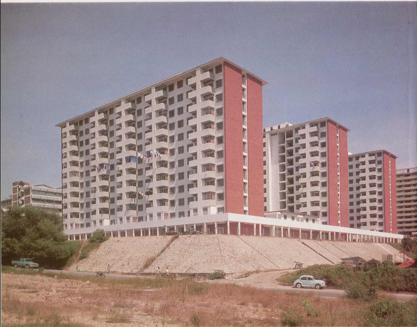
Picture shows newly completed public housing-cum-shopping complex at Chin Swee Road—part of the comprehensive redevelopment scheme, Precinct S1.
