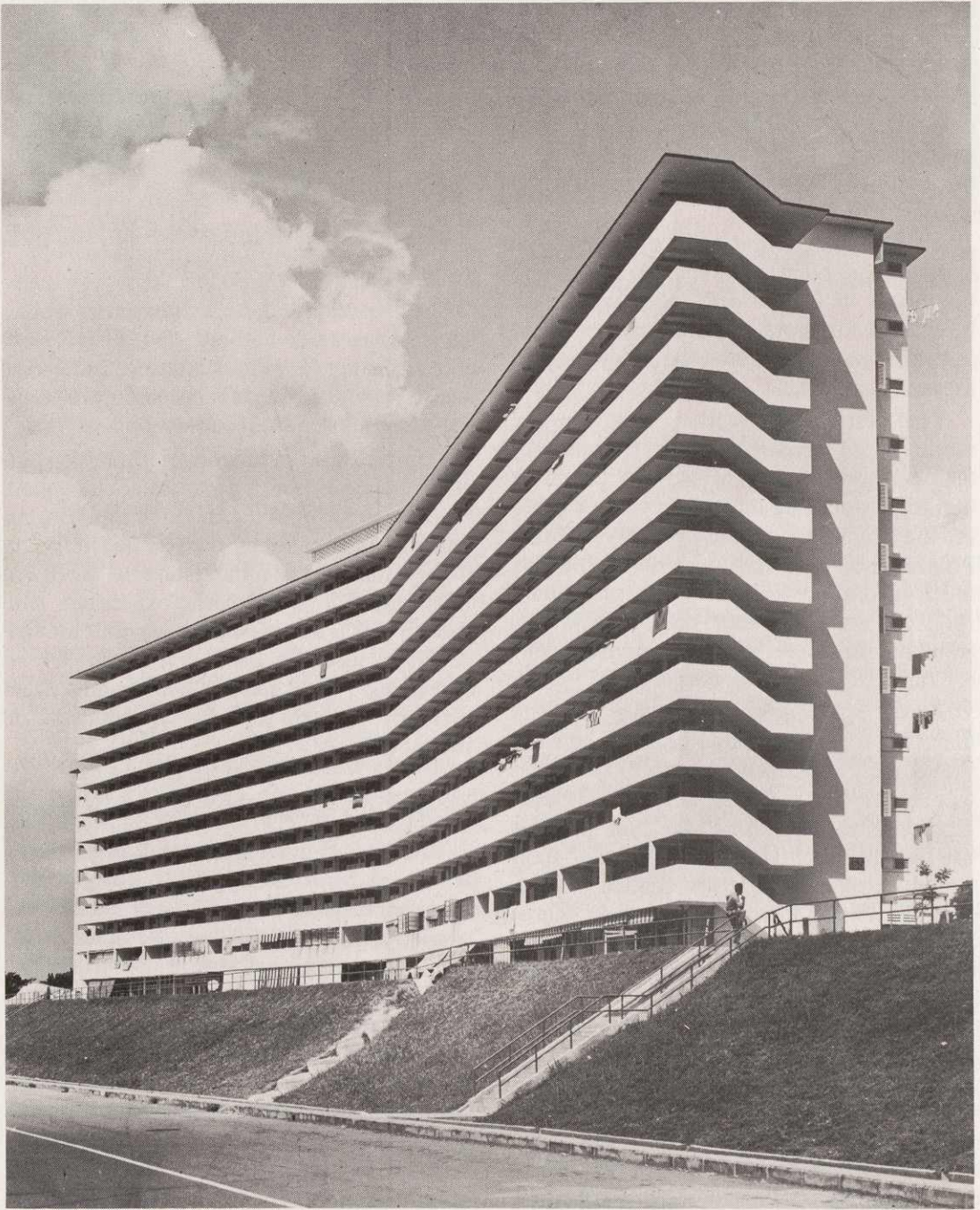
This block of 3-room Improved Flats in Toa Payoh, Neighbourhood IV is a variation from the traditional "slab" block building form.
