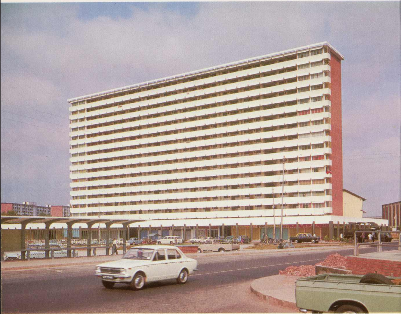
A 16-storey block of 3-room Improved flats at Margaret Drive, Queenstown, Neighbourhood II.
