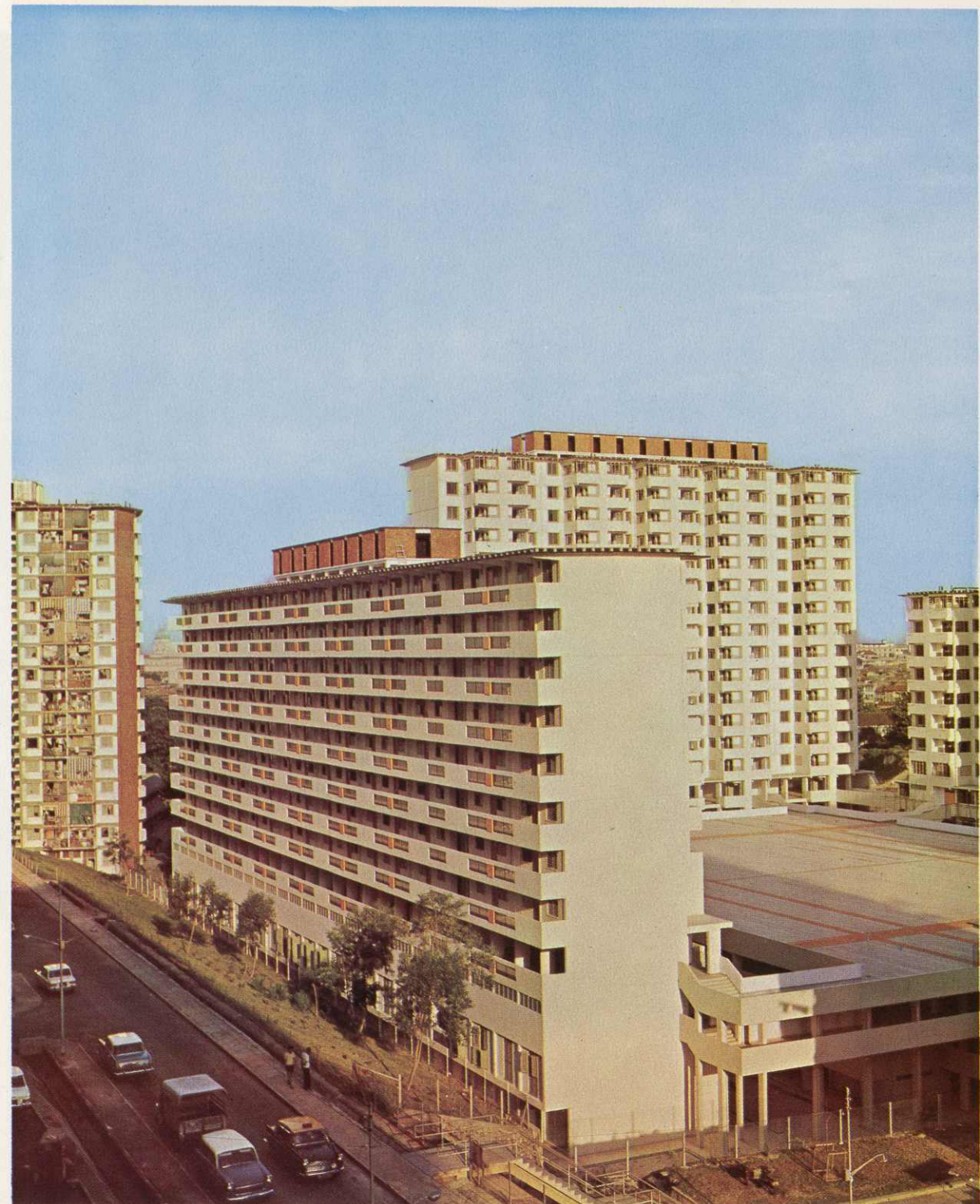
Chin Swee Road Redevelopment. This scheme comprising shops and flats, is developed under the Urban Renewal Programme. A multi-storey carpark is provided and the roof-top of the carpark serves as a recreational area for the residents.
