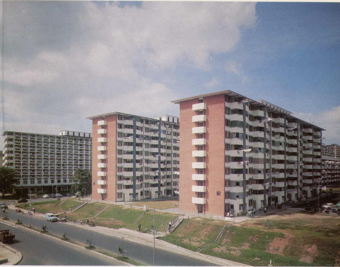
2-blocks of 1-room Improved flats at Bukit Merah Redevelopment.
