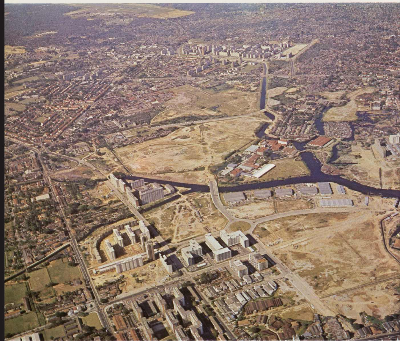
An aerial view of the Kallang Basin Reclamation and Redevelopment. About 400 acres of land have been reclaimed from the former tidal swamp. Two-thirds of the land are allocated to clean and labour-intensive industries while one-third of the land is allocated to public housing.
