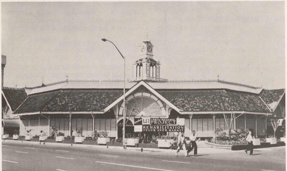
Rehabilitation of Telok Ayer Market under the Urban Renewal Programme.
