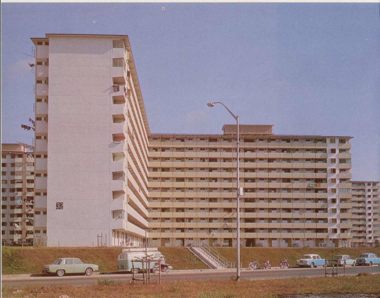
The L-shaped block of 3-room Improved Flats in Toa Payoh, Neighbourhood 1 is another variation from the traditional "Slab Block" building form.
