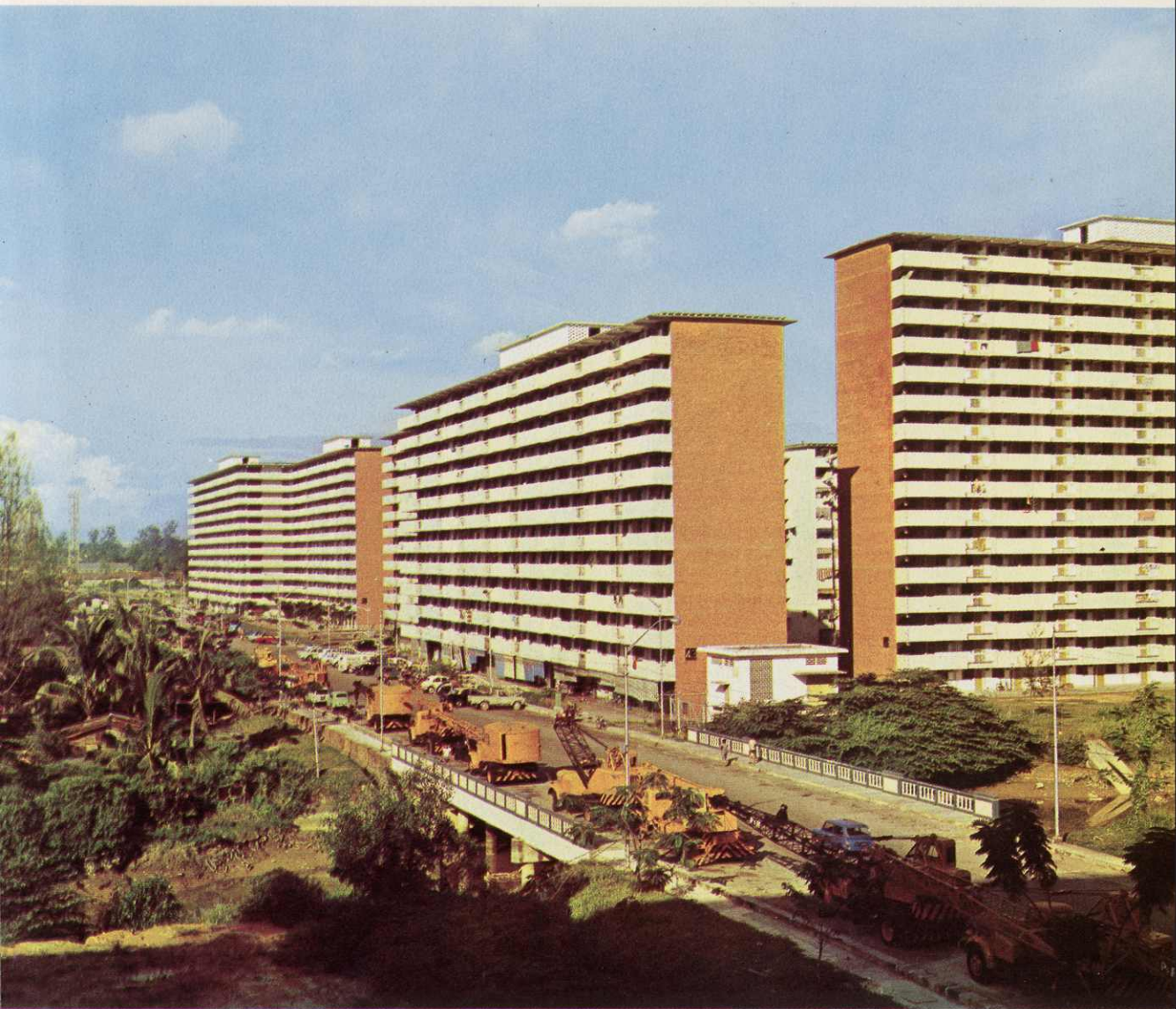
Newly completed flats in Kallang Basin, Neighbourhood II.
