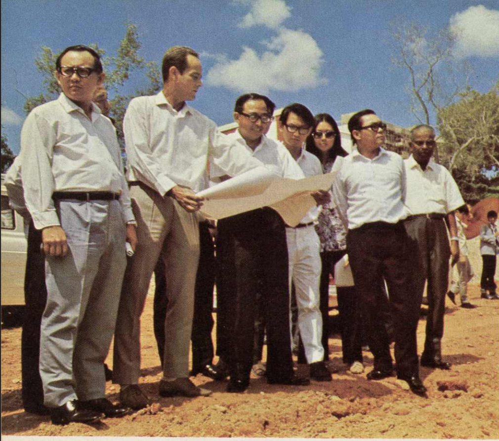
The Minister for Law & National Development, Mr. E.W. Barlow, Members of Parliament Mr. Alexendra, Ulu Pandan and Anson, Dr. Wong Lin Ken, Chiang Hai Ding, and Mr. Govindaswamy respectively, a tour of construction site accompanied by the Chairman and Chief Executive Officer.
