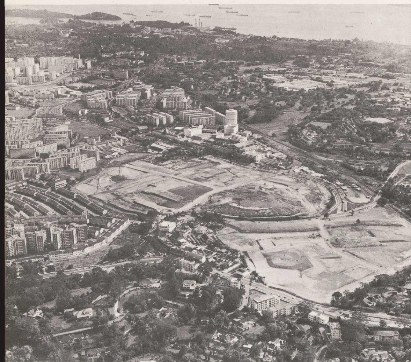
An aerial view of the completed earthworks for Queenstown, Neighbourhood VII, the last neighbourhood in the satellite town to be developed by the Board.
