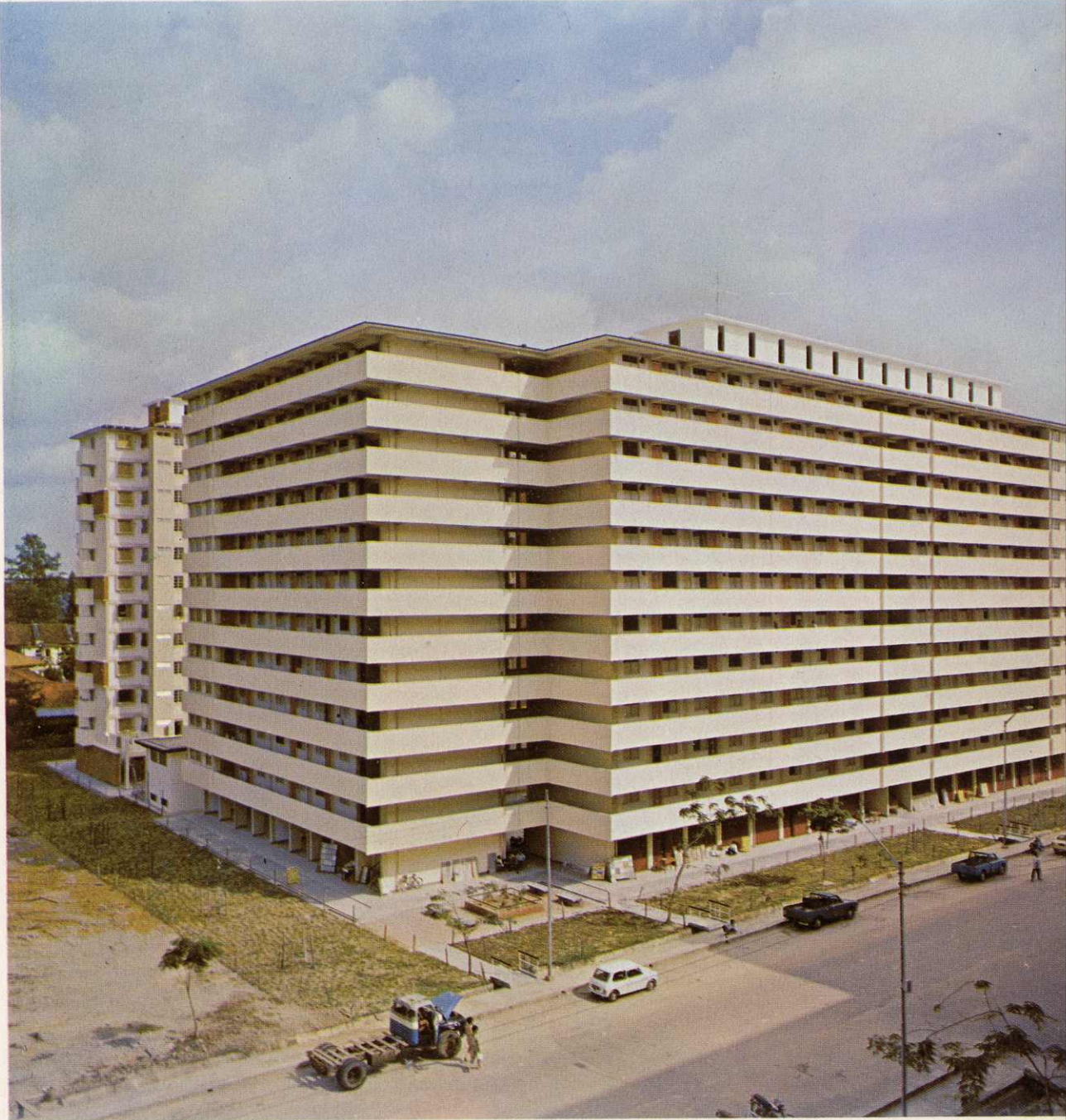
Another L-shaped 12-storey block of 3-room (Improved) flats. On the ground floor are 8 units of shops with living quarters on the first floor.
