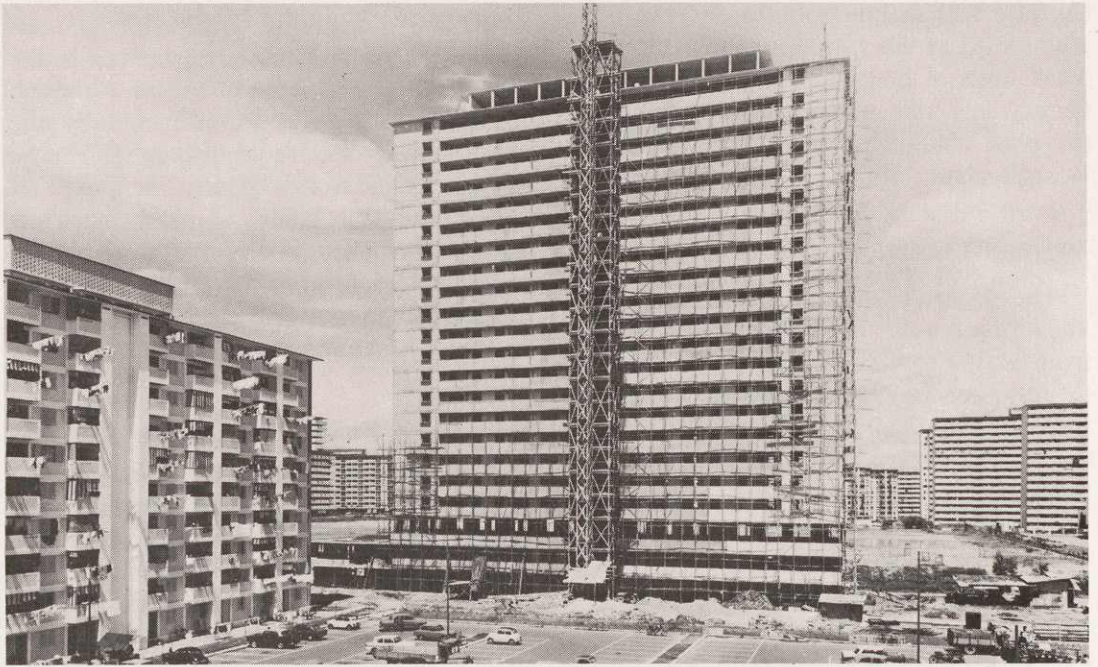
A 21-storey block under construction in Toa Payoh.
