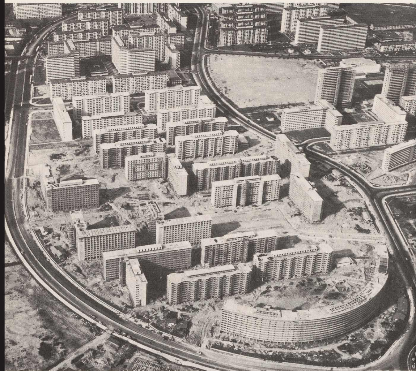
An aerial view of the buildings under construction on the southern part of Toa Payoh New Town.
