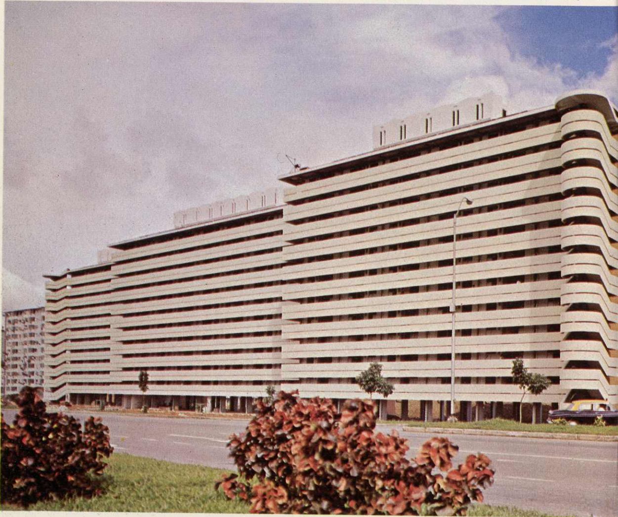
A newly completed interlinked 12-storey block of 3-room (Improved) flats in Kampong Tiong Bahru.
