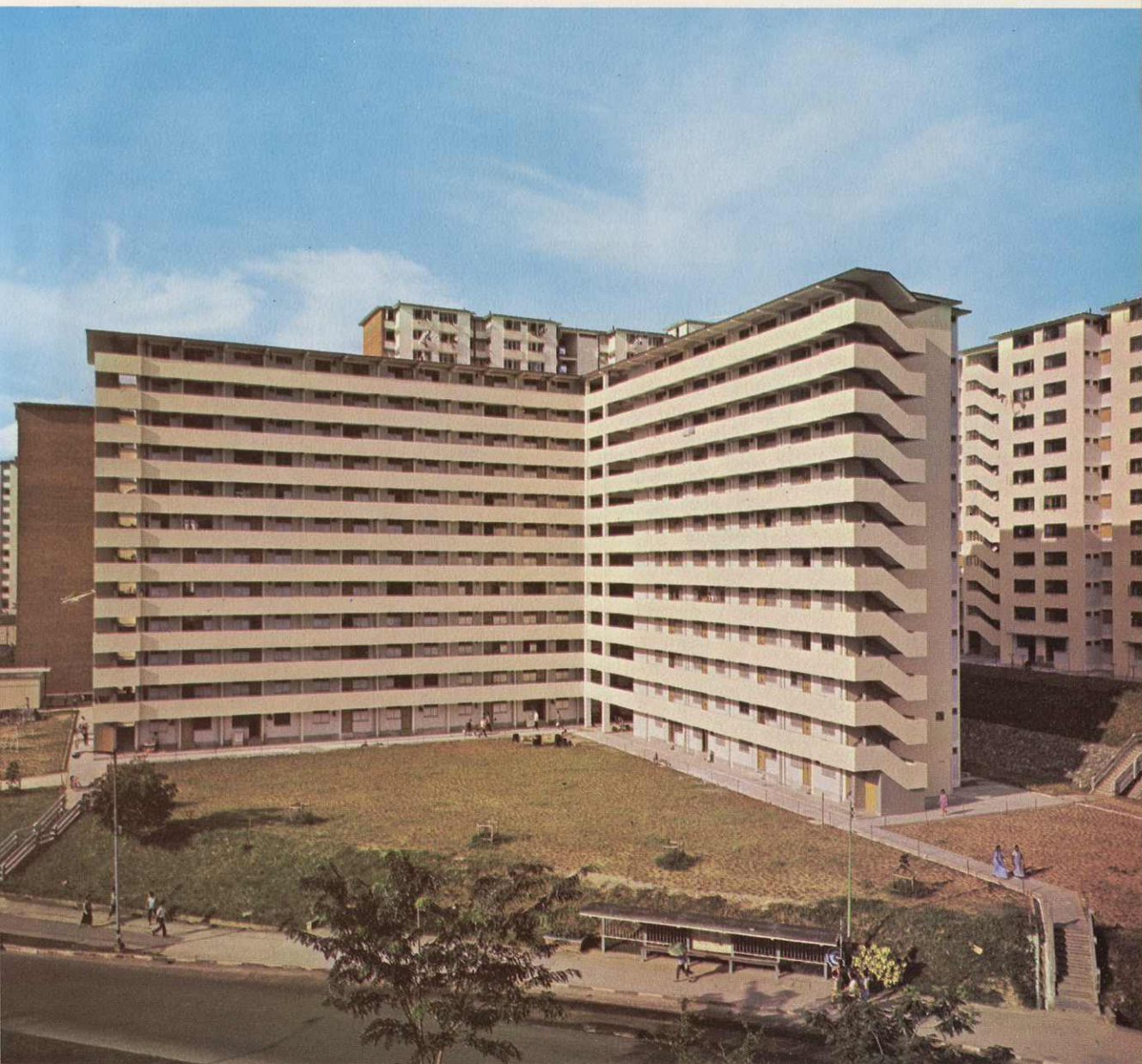
A newly completed L-shaped block of 3-room (Improved) flats in Queenstown, Neighbourhood VI.
