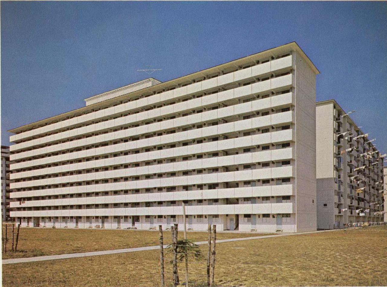
A newly designed 10-storey block of 2-room flats in Toa Payoh, Neighbourhood IV.
