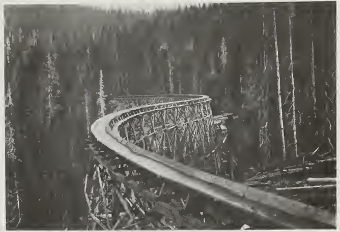
Figure 5—Trestle on French Gulch Flume 1906.
