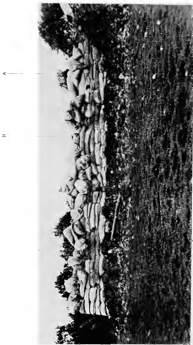
No. 2. Same parapet as in No. 1 after five minutes' alteration. Sandbags have been thrown on top. A man in a sandbag-covered helmet is looking over at A, and a man in a cap is looking between the sandbags at B. N.B.—Bags must be filled with broken stone or shingle to be bullet-proof; but should be sparsely used in case of bombardment.
