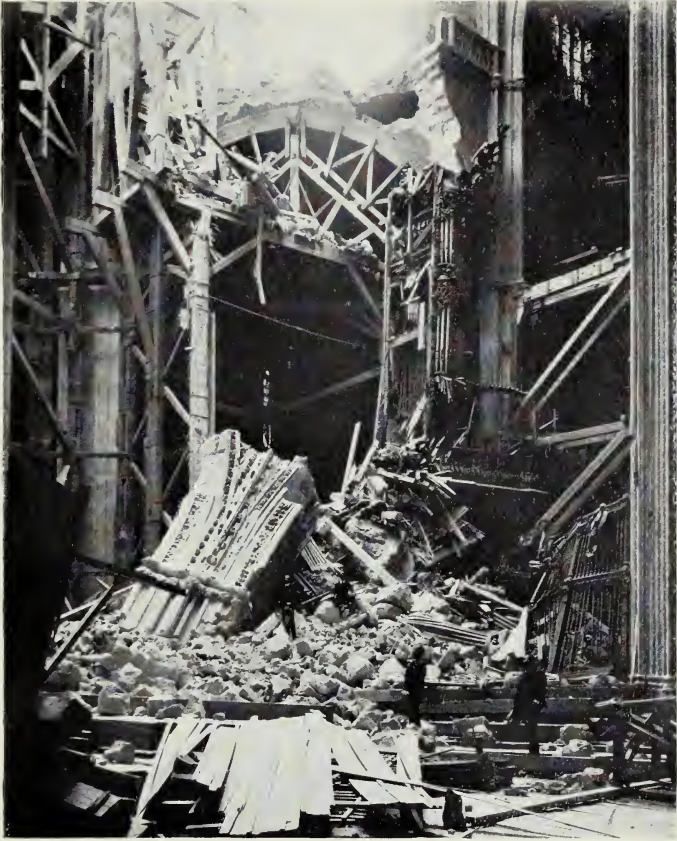
COLLAPSE OF THE CENTRAL VAULTS, SEVILLE CATHEDRAL.
