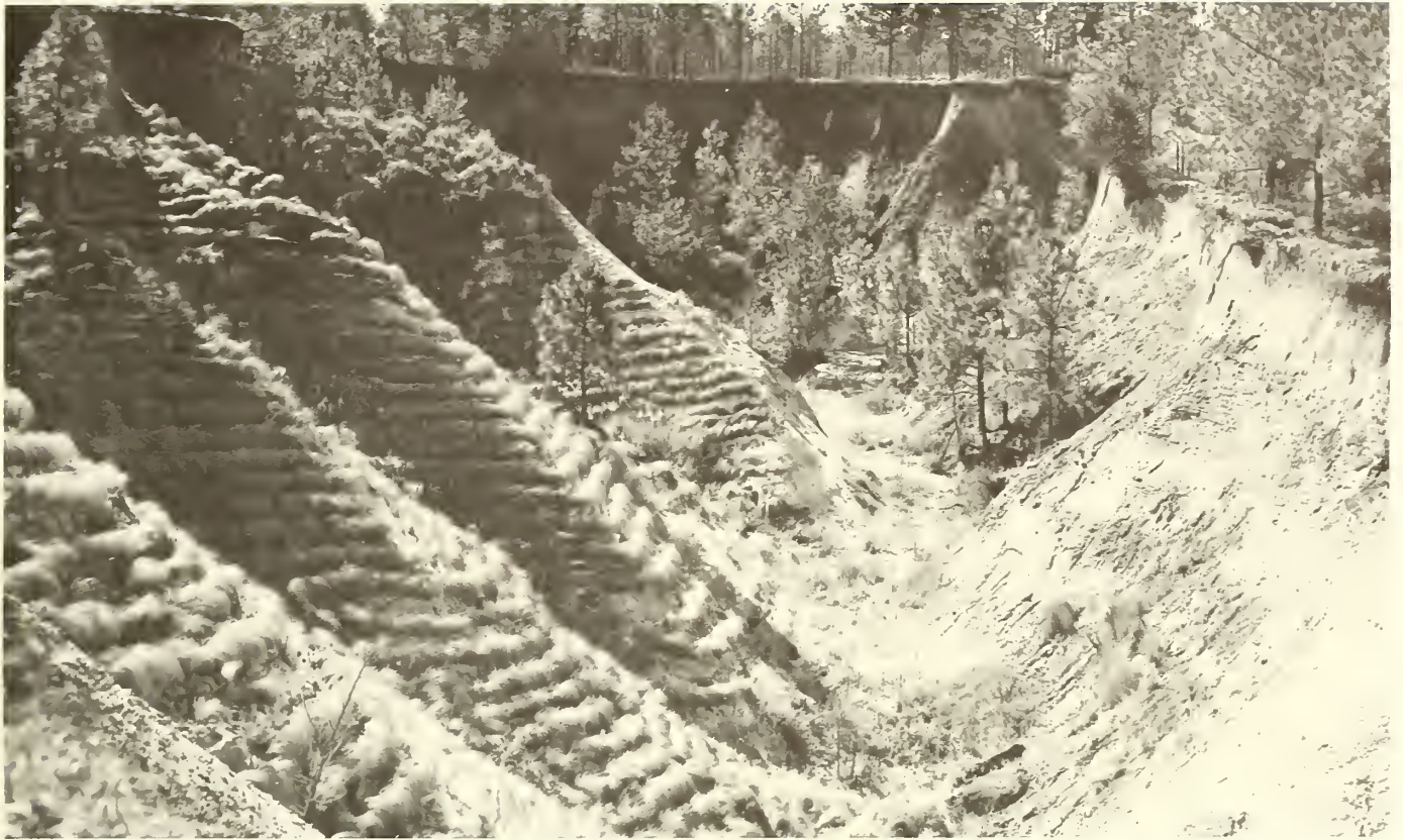
Figure 10.—Weeping lovegrass was seeded to stabilize the site prior to tree planting.
