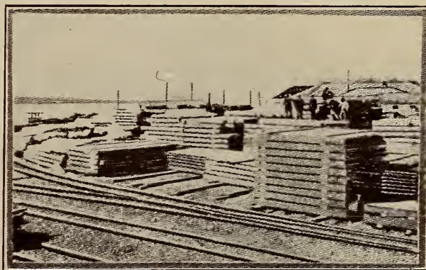
STACKS OF PINE LUMBER AT THE PORT OF PARANAGUA
