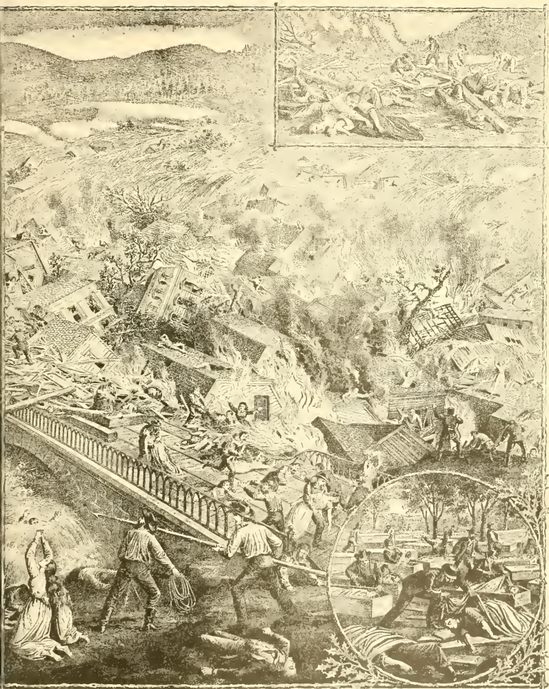
THE RAILROAD BRIDGE. N DISASTER.
