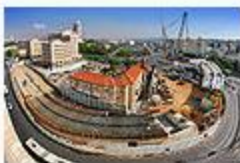
Calatrava bridge site.jpg 347 KB
