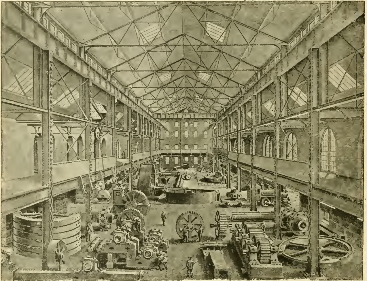
ERECTING SHOP OF THE ROBERT POOLE & SON COMPANY, BALTIMORE.
