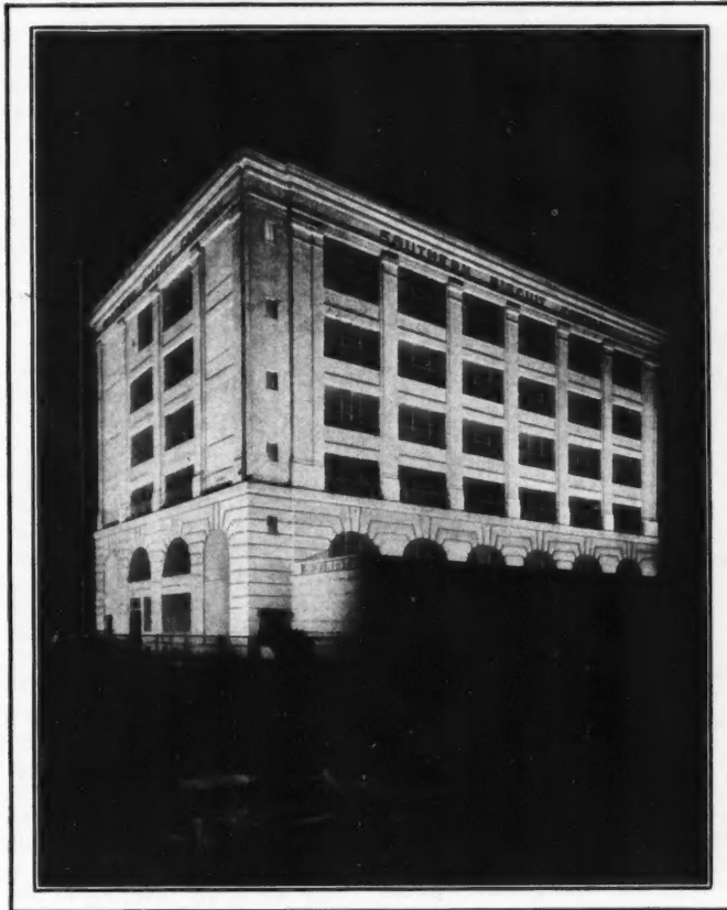
This modern factory building, the plant of the Southern Biscuit Works at Richmond, Va., demonstrates the combination of true beauty with the purely practical in reinforced concrete construction. The picture at the left shows also how splendidly a concrete exterior lends itself to flood lighting. Francisco and Jacobus, Architects, New York City.
