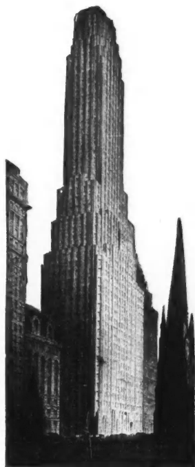
Irving Trust Company Building now being erected at One Wall Street, New York
