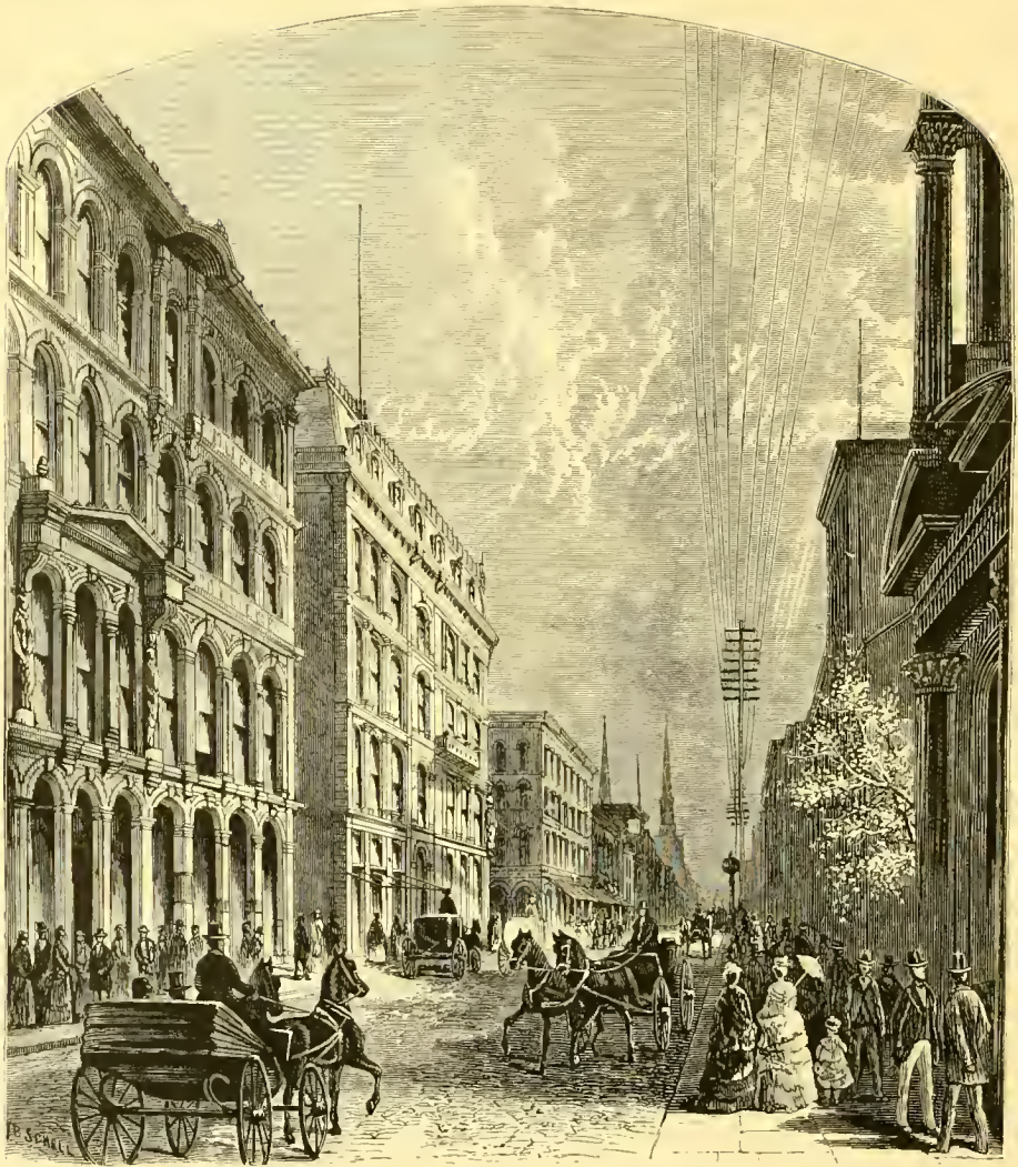
VIEW AT FIFTH AVENUE AND SIXTH STREET, PITTSBURG.
