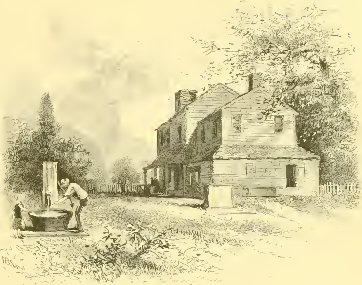
OLD HOUSE AT JAMESBURG.
