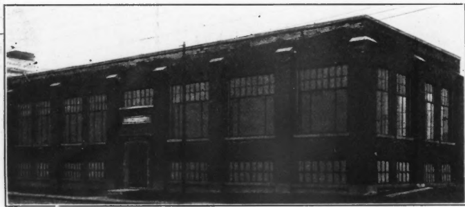
Exterior View of the Toronto Telegram's Auxiliary Plant
