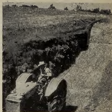
An unlined trench silo is economical to build and easily filled.
