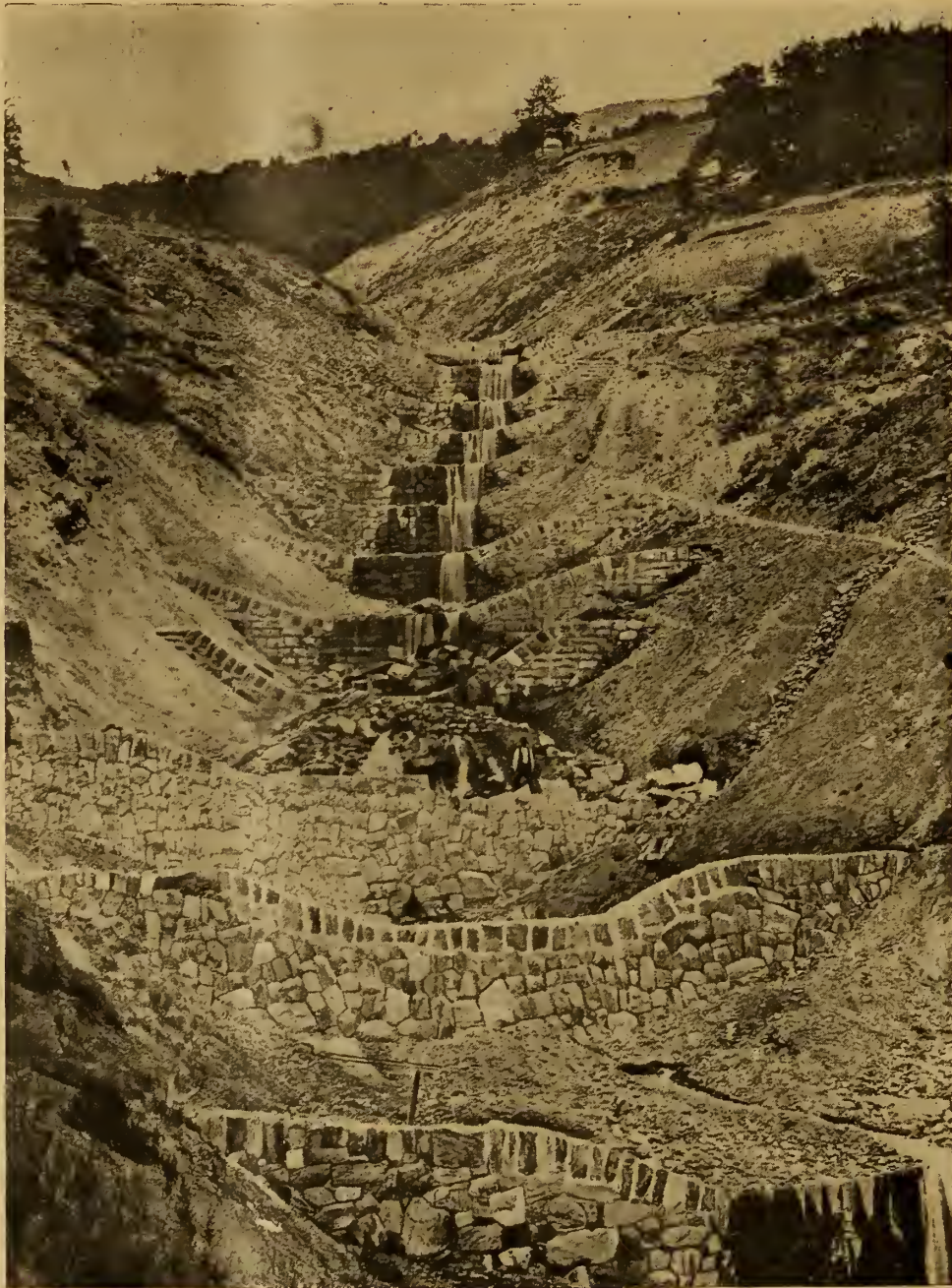
Fig. 99.—Corrective Works in one branch of the Torrent of Grollaz.—See page 621.
