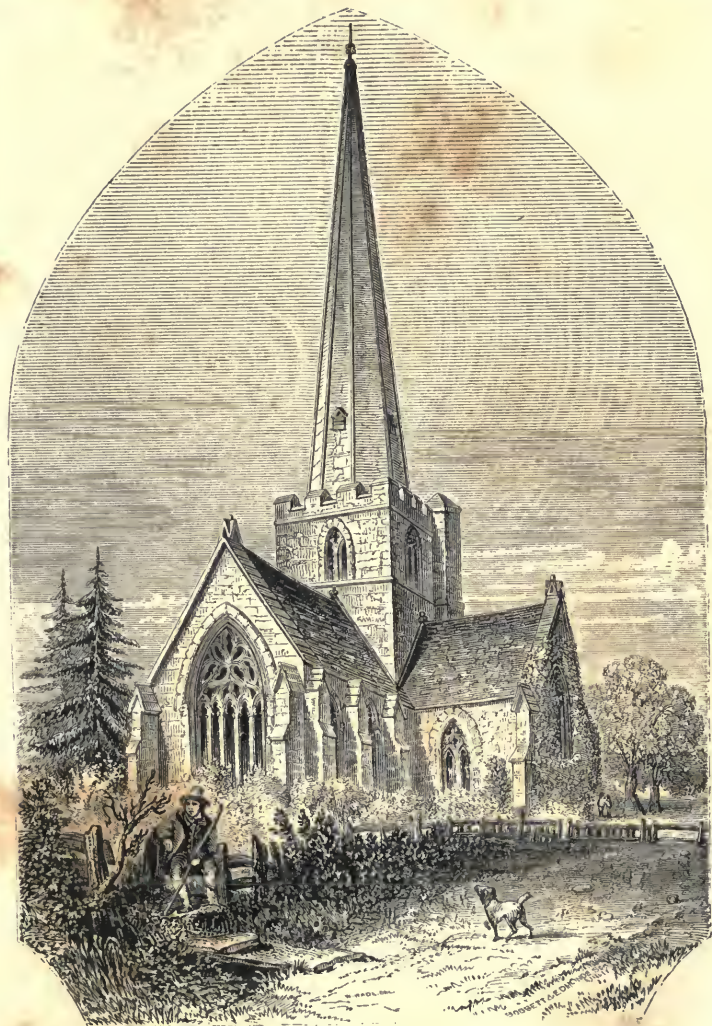
CHURCH ARCHITECTURE. (Shottesbrook Church, England.) p. 82.
