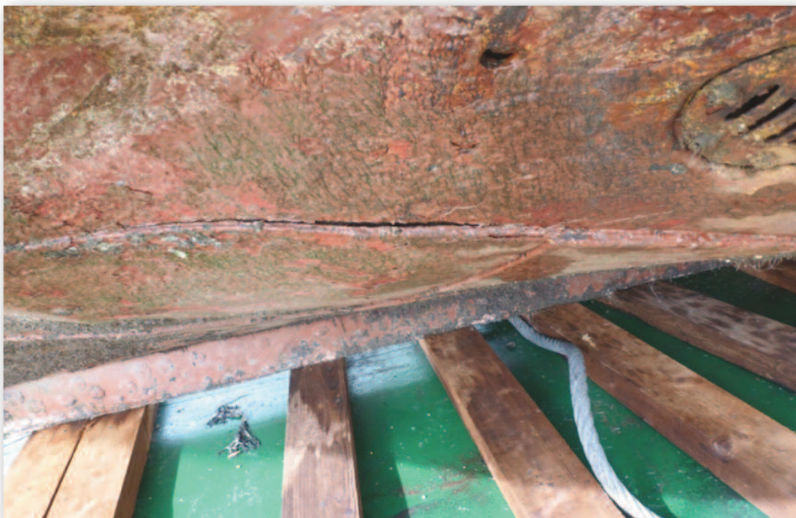
Photograph No.14 - Starboard side aft after salvage
