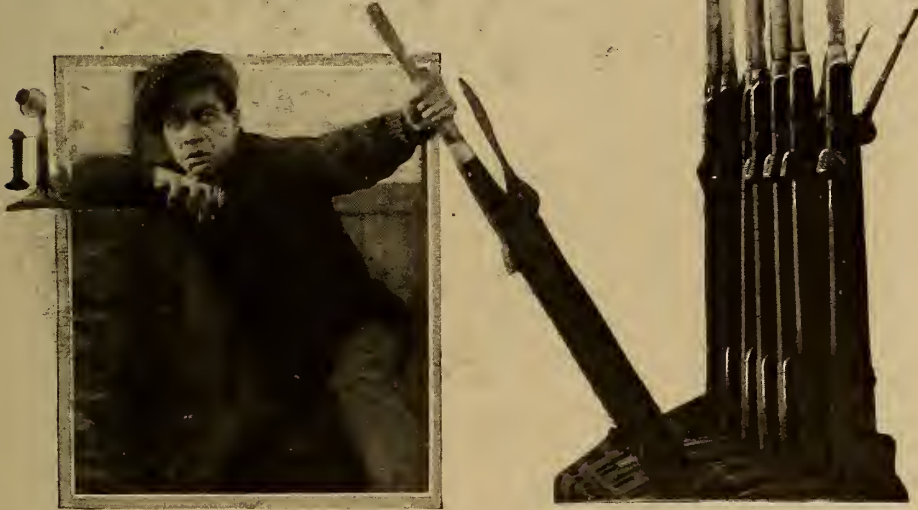
KENT SETS THE SWITCH THAT WRECKS THE EXPRESS
