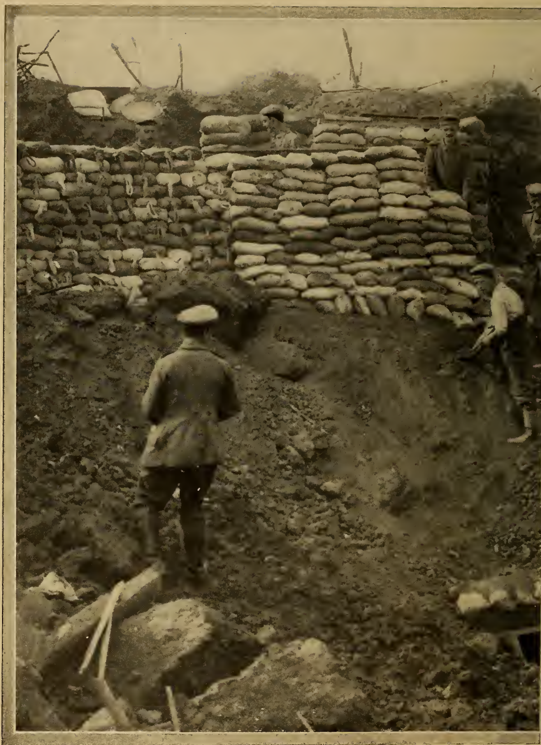
THE AUSTRIANS START TO REPAIR THE FRIGHTFUL DAMAGE
