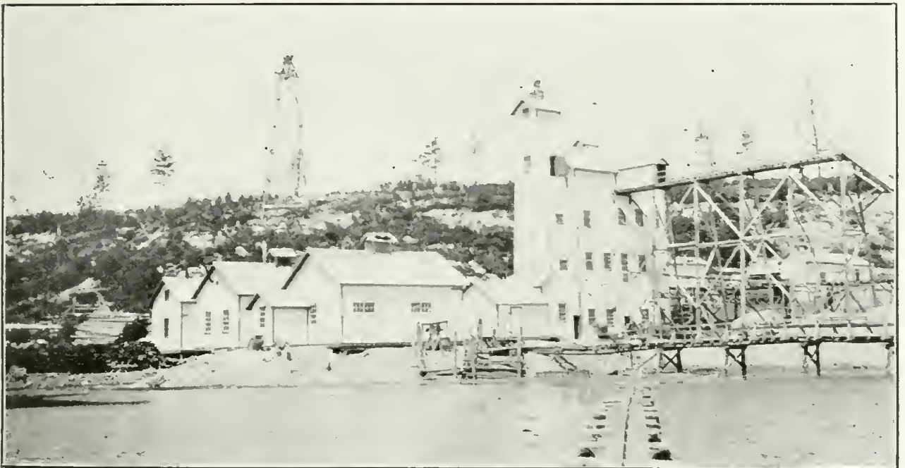
Seneca-Superior silver mine and plant.
