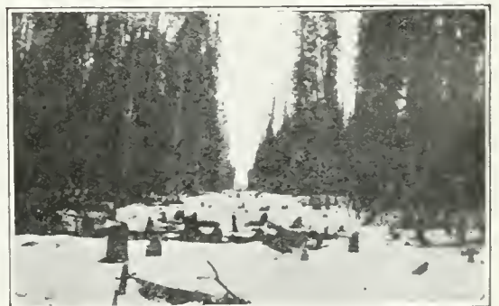
A new road on the old District boundary between Algoma and Nipissing, two miles west of the town of Cochrane.
