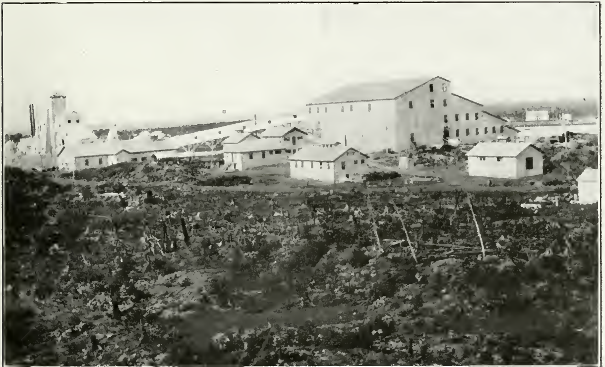
Hollinger mine, showing shaft house and mill.
