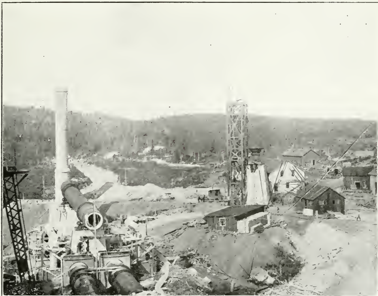
Magpie mine. showing shaft house and roasting plant in course of construction.
