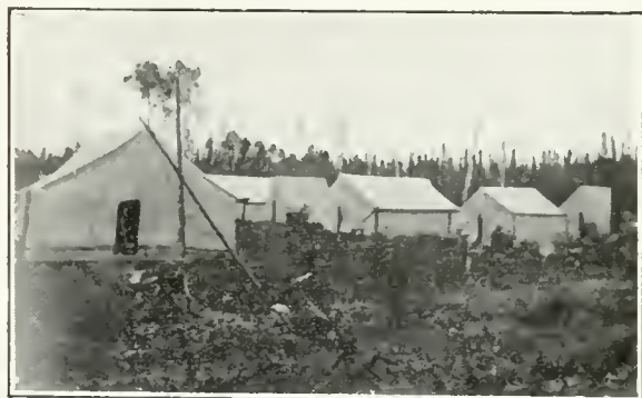
A road camp, Township of Glackmeyer.
