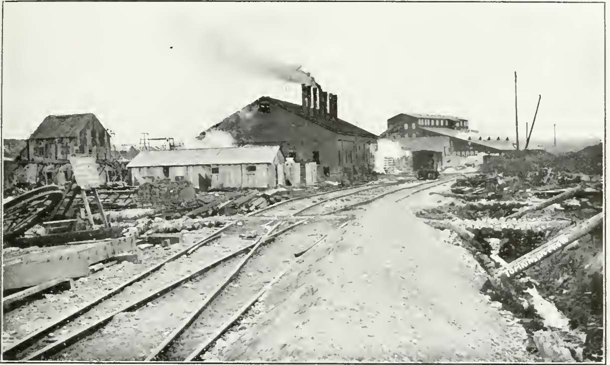
Dome mill, showing power house and mill.
