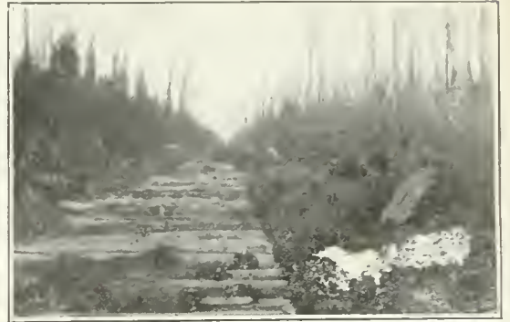
An unfinished corduroy road through semi-muskeg land.
