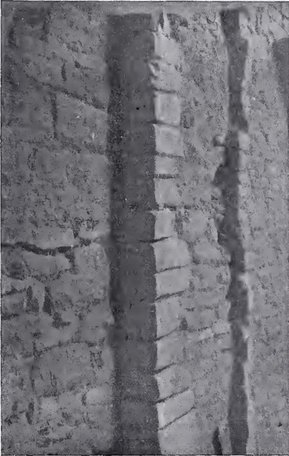
WINTERTON CHURCH TOWER. DETAILS OF EARLY MASONRY ON SOUTH SIDE.
