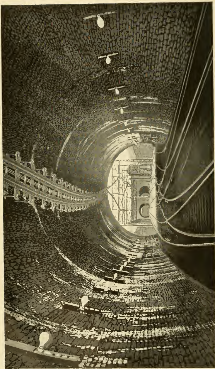
LOOKING OUT THE BREVORT STREET PORTAL OF THE BELT LINE TUNNEL, BALTIMORE—THE LARGEST TUNNEL OPENING IN THE WORLD. TRAINS ARE DRAWN THROUGH THIS TUNNEL BY ELECTRIC ENGINES.
