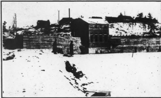
POWER PLANT OF THE PENN IRON MINING COMPANY
