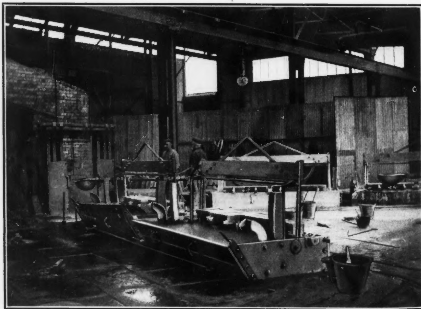
LADLE ON TRAVELING CARRIAGE AND WATER TANKS, RIO TINTO REFINERY
