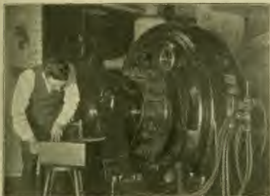
INSPECTOR MAKING MEGGER TEST ON D. C. GENERATOR TO DETERMINE CONDITION OF INSULATION.
