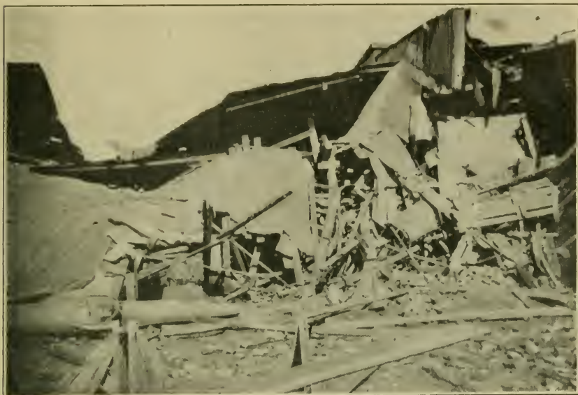
Excessive internal corrosion in a horizontal tubular boiler at a brick yard in Richmond, Va., caused the explosion shown above. The accident demolished the building and wrecked an engine, causing property damage of almost $10,000.
