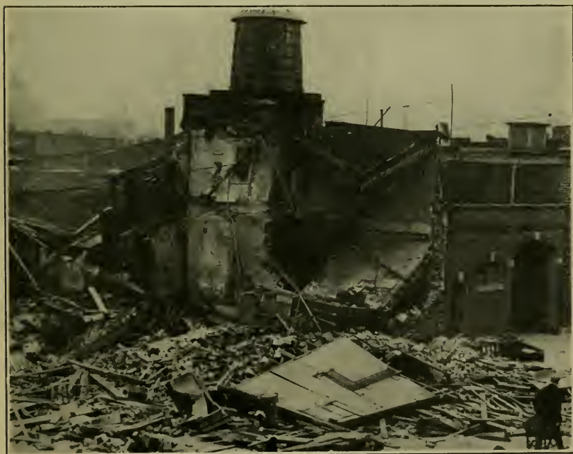
AMMONIA GENERATOR EXPLOSION AT PHILADELPHIA, PA.
