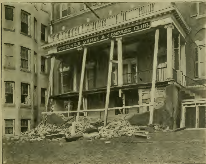
HOT WATER SUPPLY TANK EXPLOSION AT WORCESTER, MASSACHUSETTS
