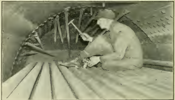
EXAMINING THE INSIDE OF A BOILER.
