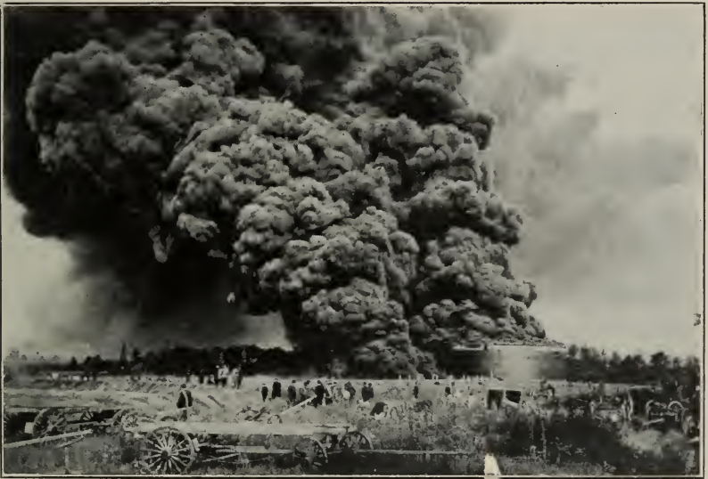
A 35,000-barrel tank fire.
