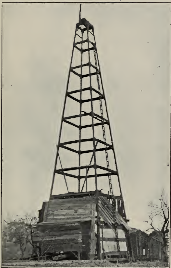
The steel derrick.
