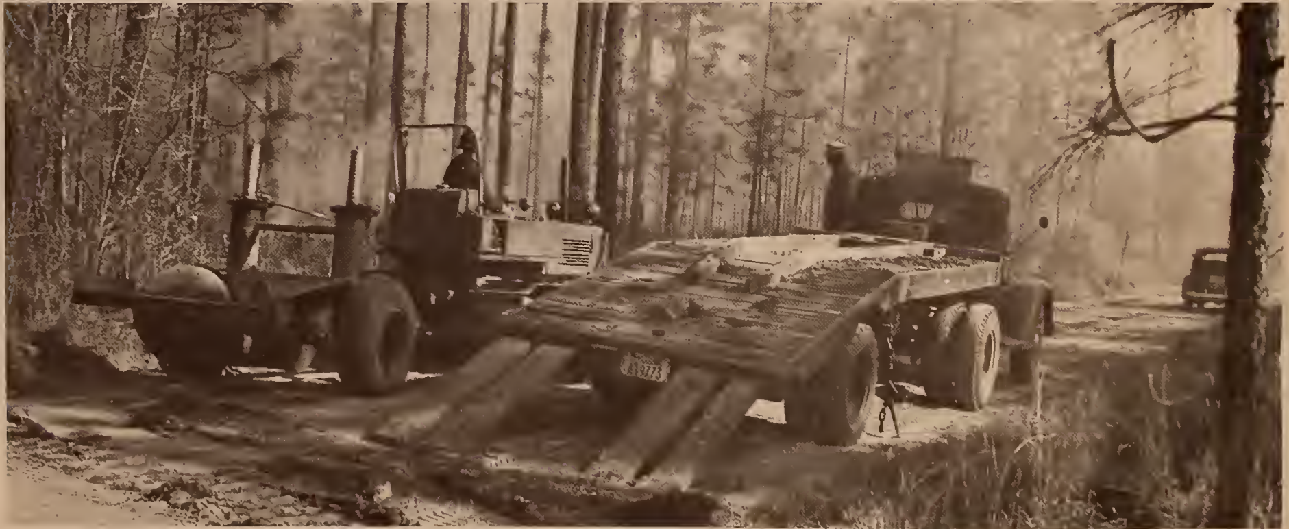
Fire-line plow ready to roll, on a Francis Marion fire.
