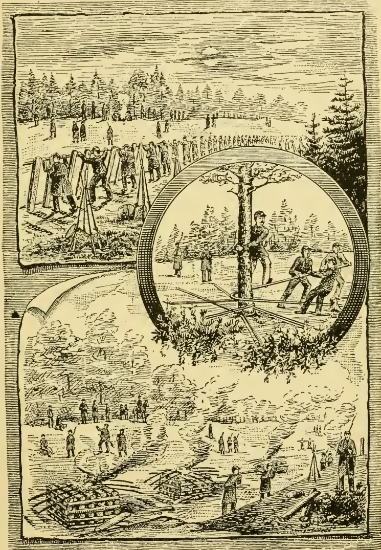
TEARING UP THE WELDON RAILROAD.
