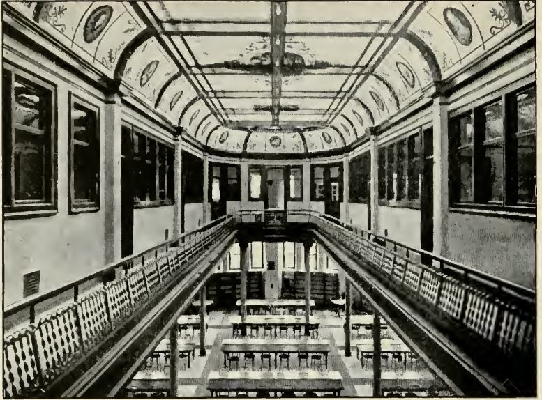
THIRD FLOOR BALCONY AROUND SKYLIGHT OPENING To the Main Reading Room below. Showing Subskylight, Doors and Inner Windows to Seminar Rooms on Sides and End
