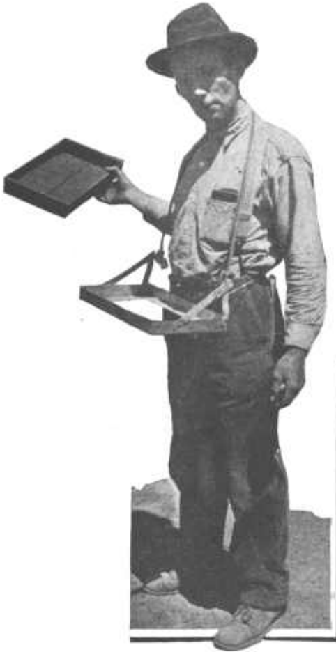
FIGURE 13.—A waist carrier designed to hold a tray used in picking blackberries
