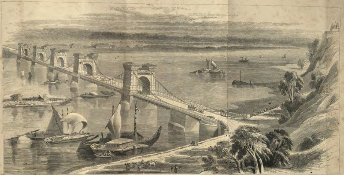
365. CL. VII., 105.—MODEL OF THE WROUGHT-IRON BAR CHAIN SUSPENSION BRIDGE AT KIRKP, NOW ERECTING ACROSS THE DISTRICT, DESIGNED BY CHARLES FENOLLE, TRAFALGAR SQUARE.
