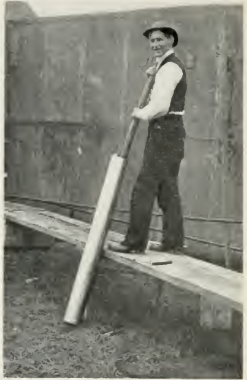
Fig. 37—LOADING A SHELL WITH SOLIDIFIED NITROGLYCERIN
