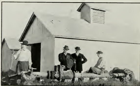
Fig. 150—TESTING A LARGE CAPACITY METER IN THE FIELD
