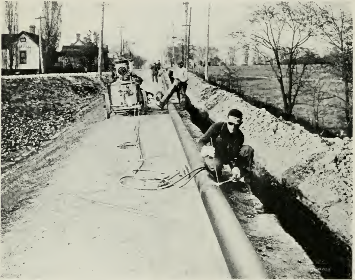
Fig. 165—WELDING LOW PRESSURE MAINS
