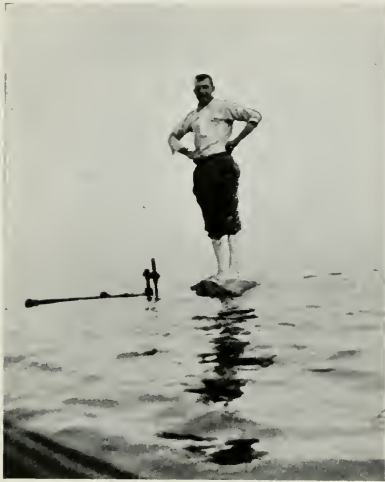
Fig. 28—GAS WELL IN LAKE ERIE Located about one-half mile from shore in twelve feet of water. Concrete pier is hardly visible above water level. Note lead line from well just level with water.
