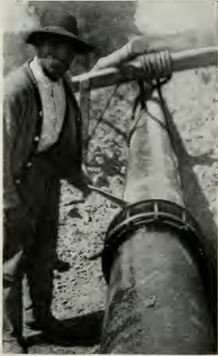
Figs. 90 and 91—"WRENCHING UP" PLAIN END CENTER RINGS
