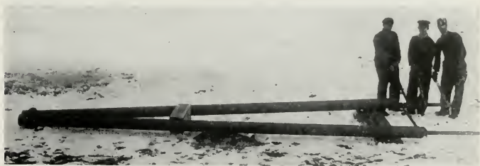
Fig. 86—MAKING FIRE BEND
