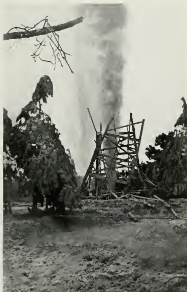
Fig. 26—A BLOWOUT IN GOOSE CREEK FIELD (TEX.)
