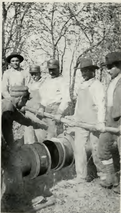
Fig. 89—STABBING PLAIN END PIPE
