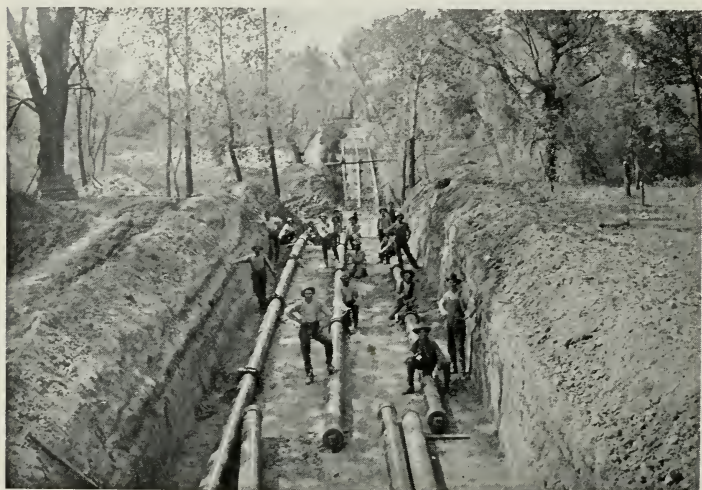
Fig. 76—RIVER CROSSING SHOWING TRIPLE LINES
