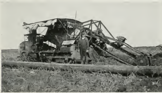
Fig. 65—DITCHING MACHINE AT WORK FOR A HIGH PRESSURE GAS LINE
