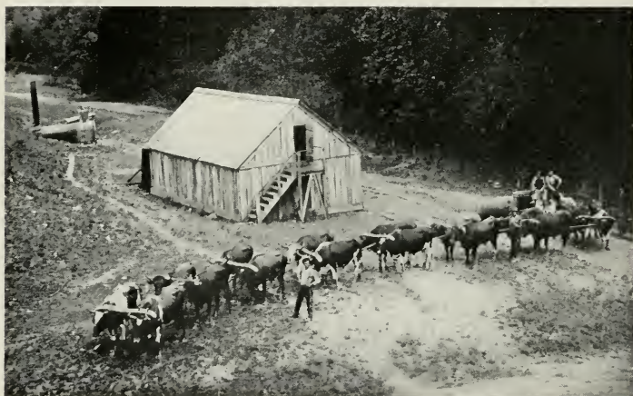
Fig. 14—MOVING A DRILLING BOILER WITH OXEN IN BLUE CREEK FIELD (W. VA.)
