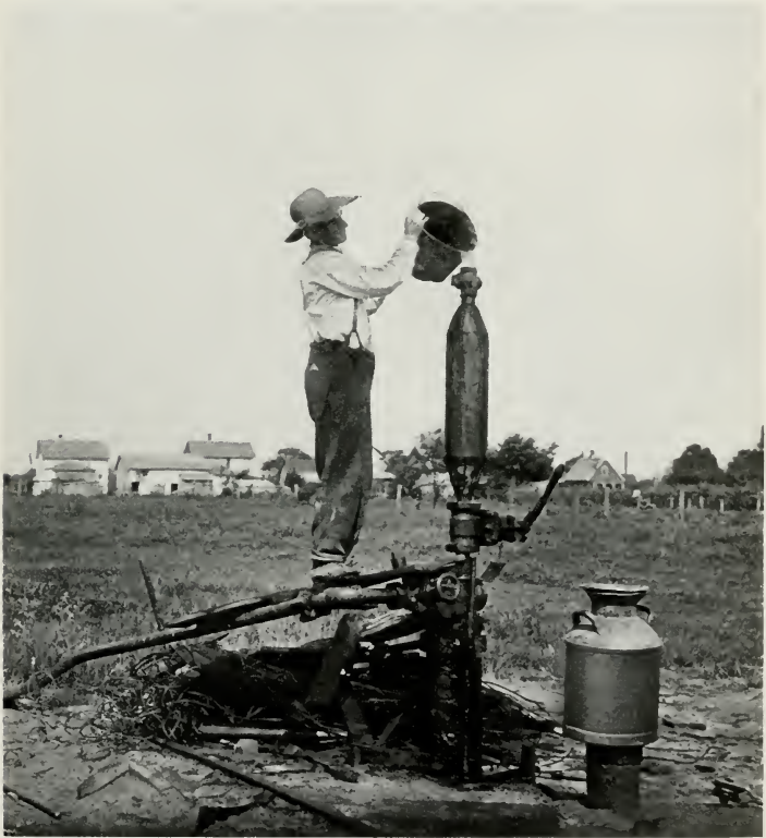
Fig. 57—WATERING A GAS WELL
