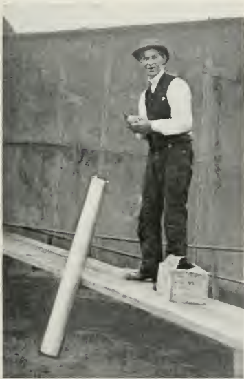
Fig. 36—PREPARING SOLIDIFIED NITROGLYCERIN TO LOAD INTO SHELL FOR SHOOTING GAS WELL
