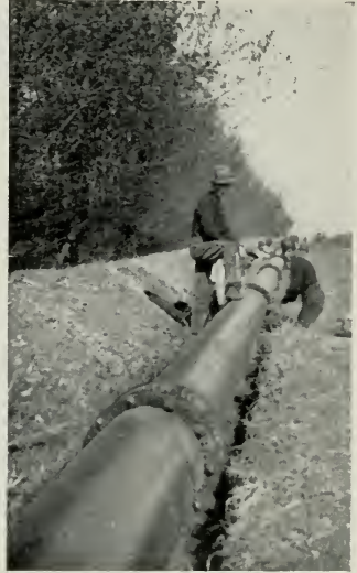
Figs. 90 and 91—"WRENCHING UP" PLAIN END CENTER RINGS
