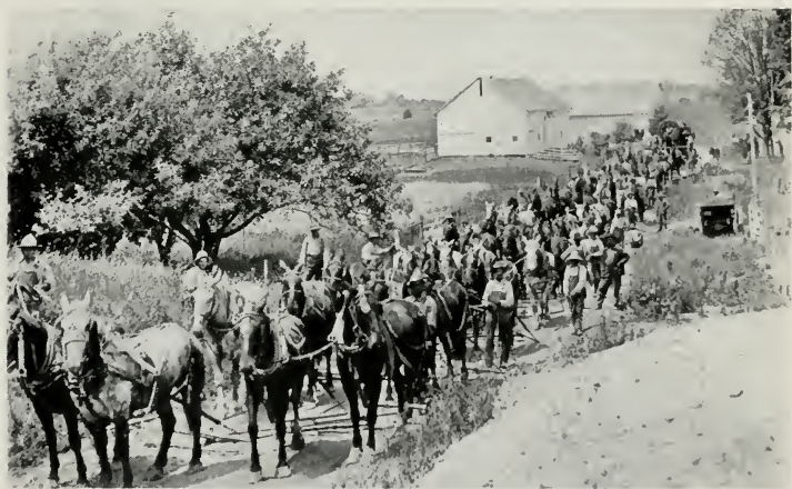
Fig. 122—HAULING A COMPRESSOR BED FROM RAILROAD TO COMPRESSOR PLANT
