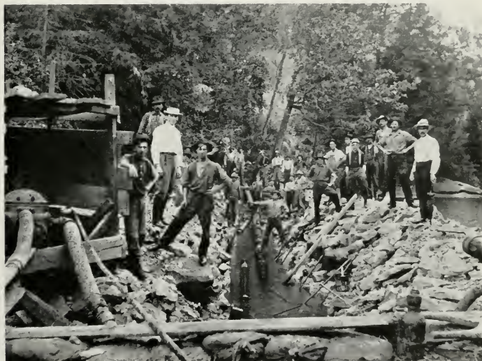
Fig. 112—LAYING 6 \frac{5}{8} " HIGH PRESSURE GAS LINE ACROSS THE MIDDLE FORK RIVER, BARBOUR CO., W. VA. Line is Being Laid in Bed of River.
