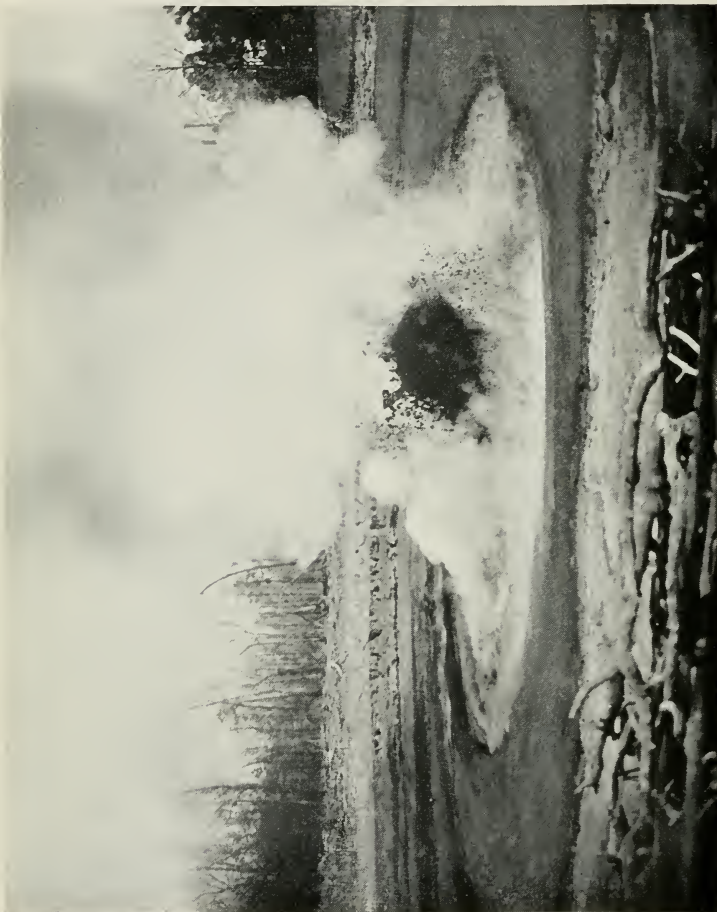
Fig. 24—THE BURNING WELL AT MOORINGSPOUT, L.A., 1912. Showing crater formed by gas "blowing out" around casing Width of the crater was about 500 feet
