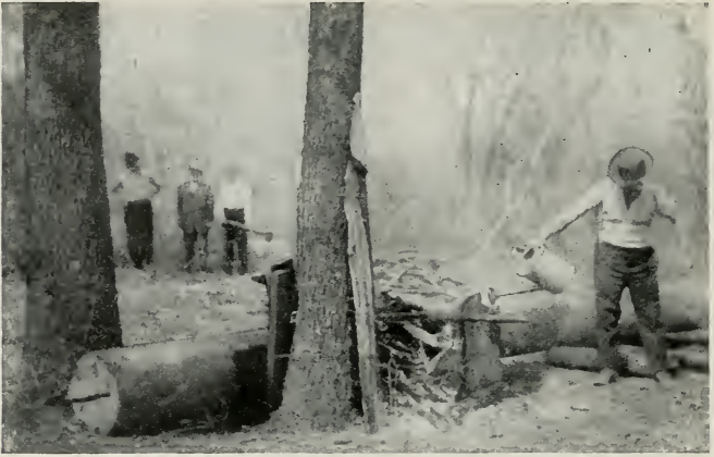
Fig. 87—BENDING JOINT OF 16-IN. PIPE BY FIRE METHOD OR HEATING
