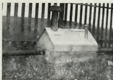
Fig. 161—SHEET IRON HEATER FOR GAS LINE
