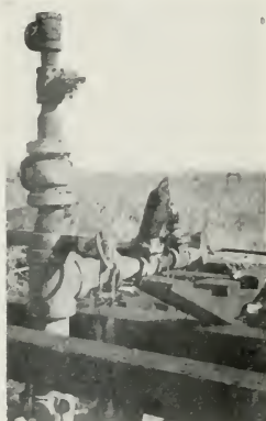
Fig. 143 The "Burning Well" at Caney, Kans., (1909) after it was capped and shut in.
