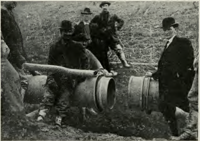
Fig. 88—PLAIN END PIPE READY TO STAB
