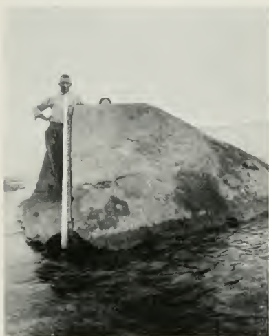
Fig. 29—GAS WELL IN LAKE ERIE
