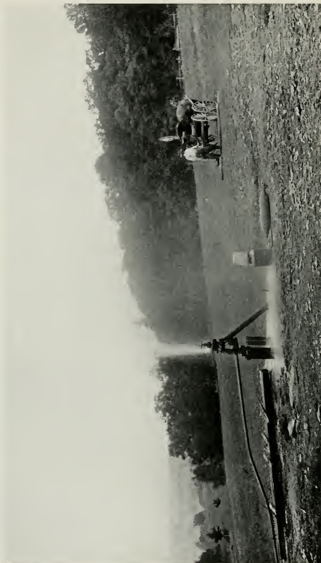
Fig. 58—SWABBING A GAS WELL
