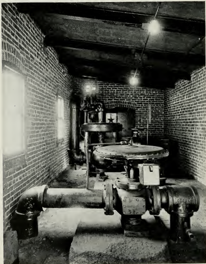
Fig. 162—LOW PRESSURE REGULATOR INSTALLATION Note Single and Double Diaphragm Regulators
