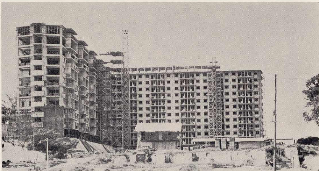
Construction of buildings at Ban Kee site of Precinct South I.
