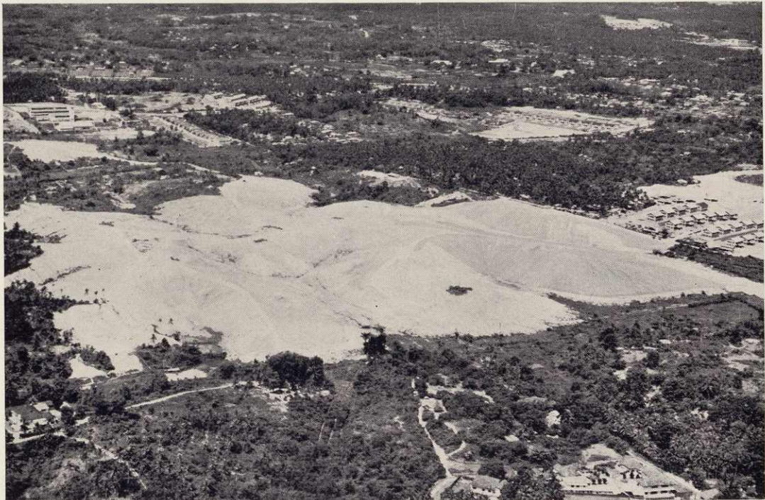
Earth excavated from the hills at Changi and Bedok is being used for the East Coast Reclamation.
