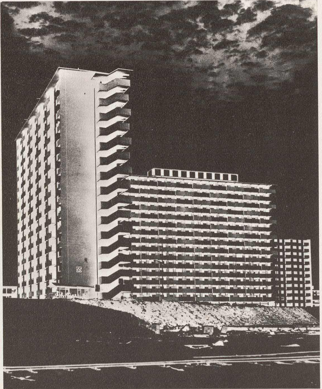
A 16-storey L-shaped building at Redhill Extension Estate.
