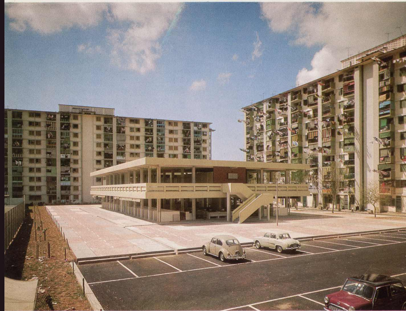
A 2-storey hawker centre recently completed in Tanjong Rhu Estate.
