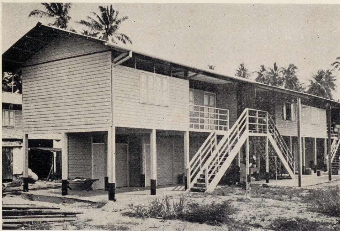
(10) Close-up view of terrace houses at Koh Seck Lim Road.
