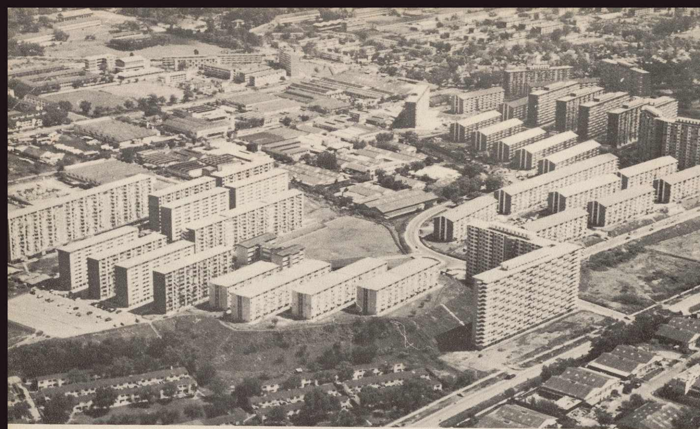
Aerial view of Alexandra Hill Estate and Redhill Extension.
