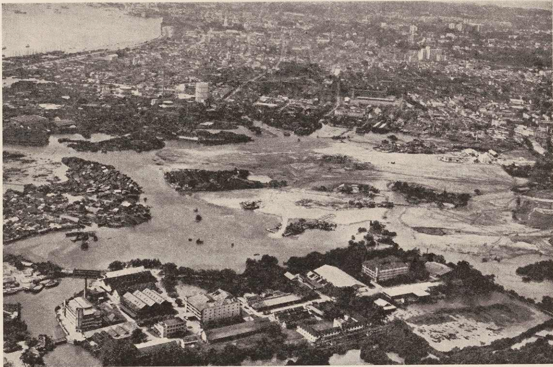
Reclamation work at Kallang Basin. Area already reclaimed is at centre and right of centre.
