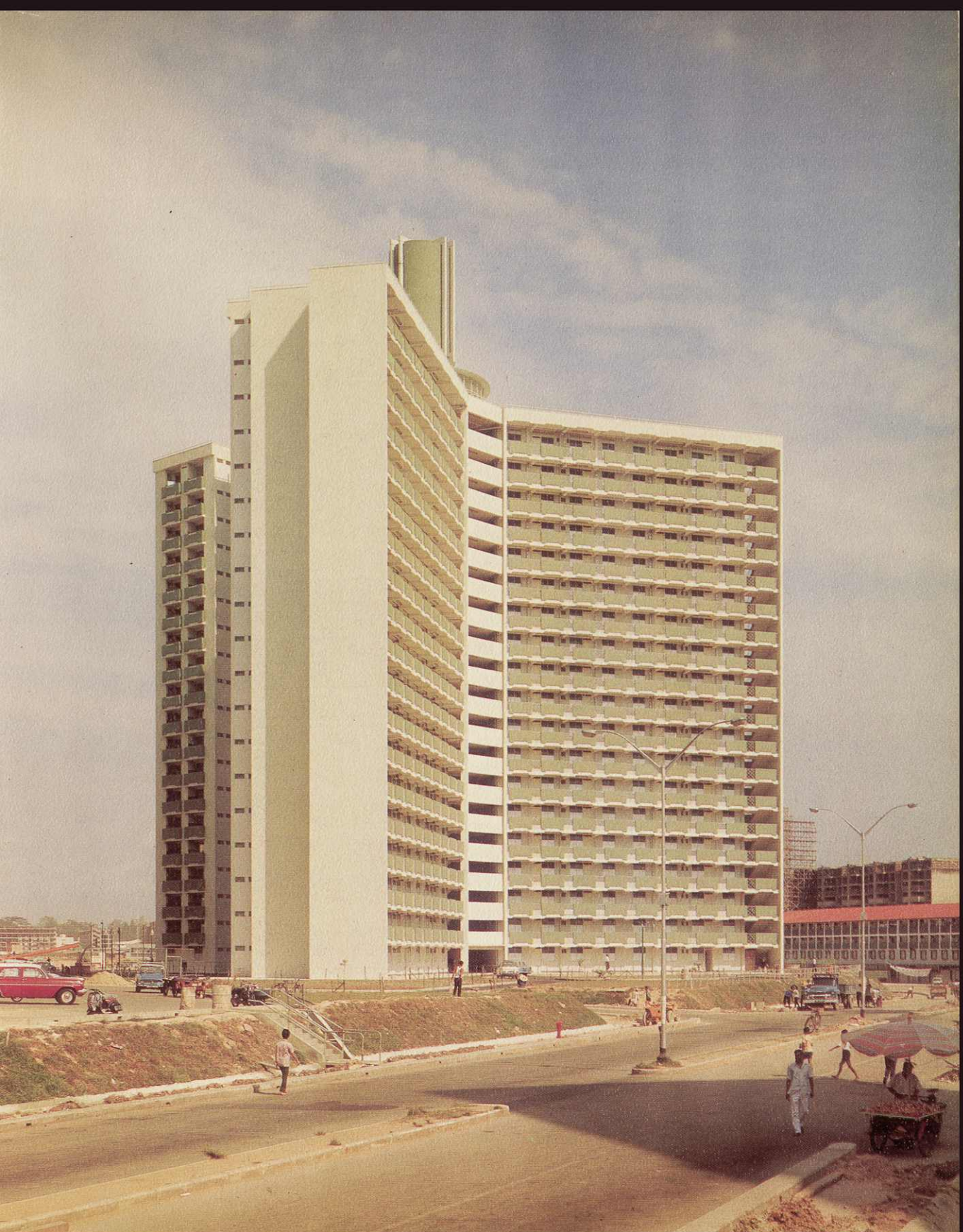
19-storey Y-shaped block (improved 3-room flats) at Toa Payoh Estate, sold under the "Home Ownership for the People" Scheme. The selling price for a 3-room flat of 650 sq. ft. of internal area is $7,500/-. (Singapore $3.02 = US $1)
