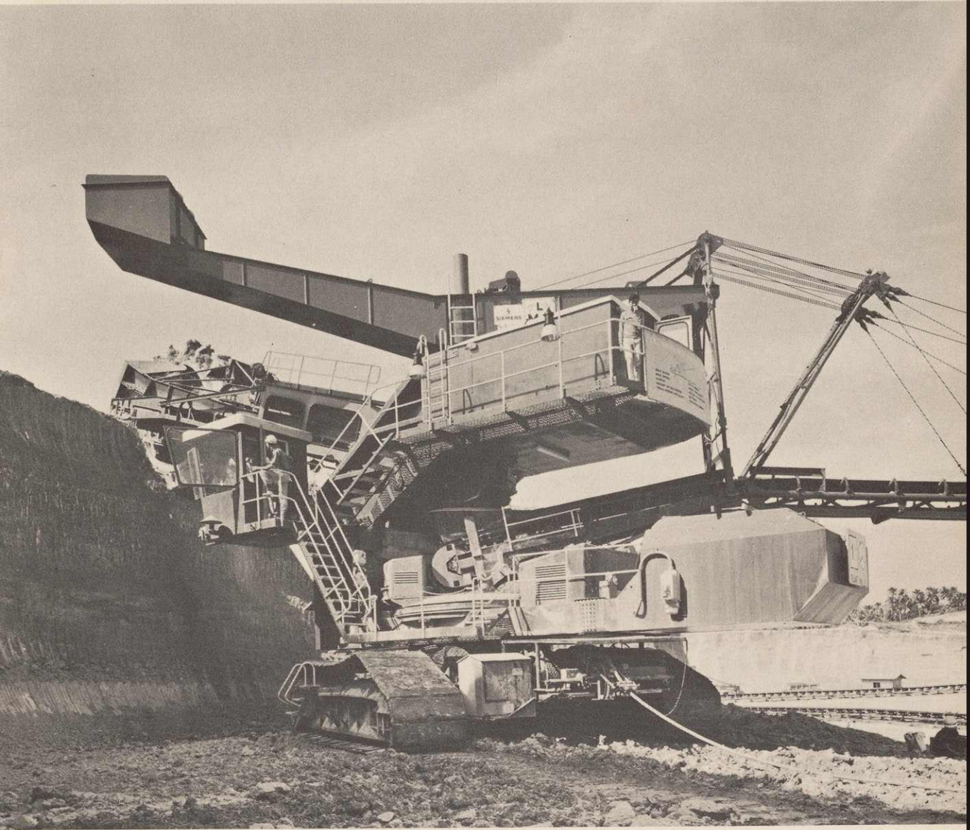
A bucket wheel excavator excavating earth at Bedok Plain.
