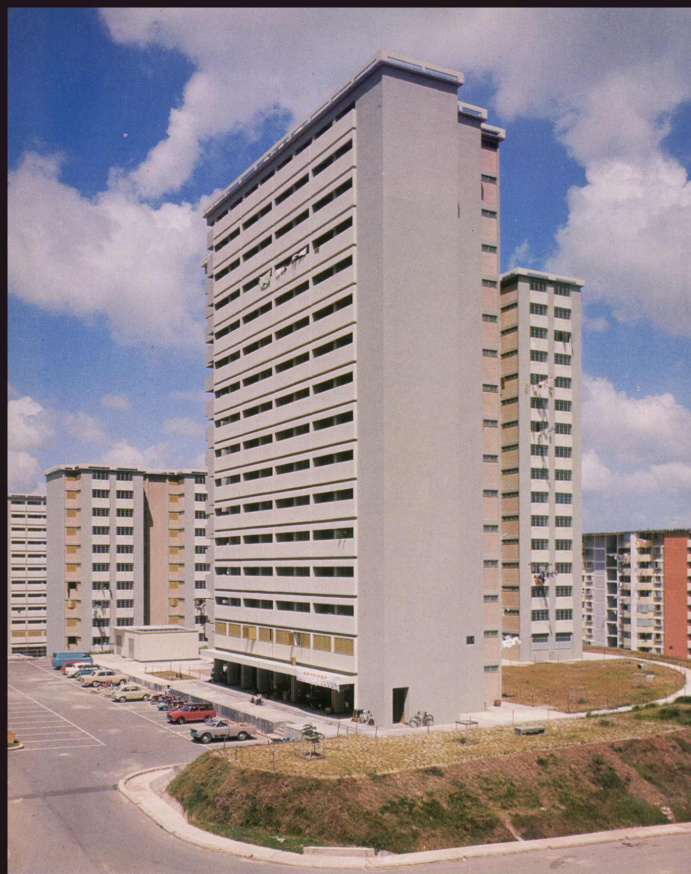
A closer look at a block of multi-storey flats at Neighbourhood 6, Queenstown, sold under the "Home Ownership for the people" Scheme.
