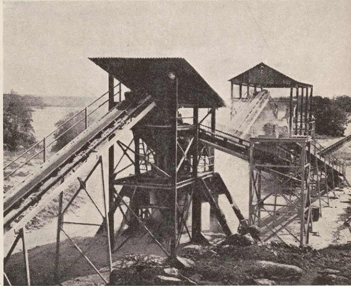
Pulau Ubin Quarry in operation. The quarry produces about 10,000 tons of granite per month.
