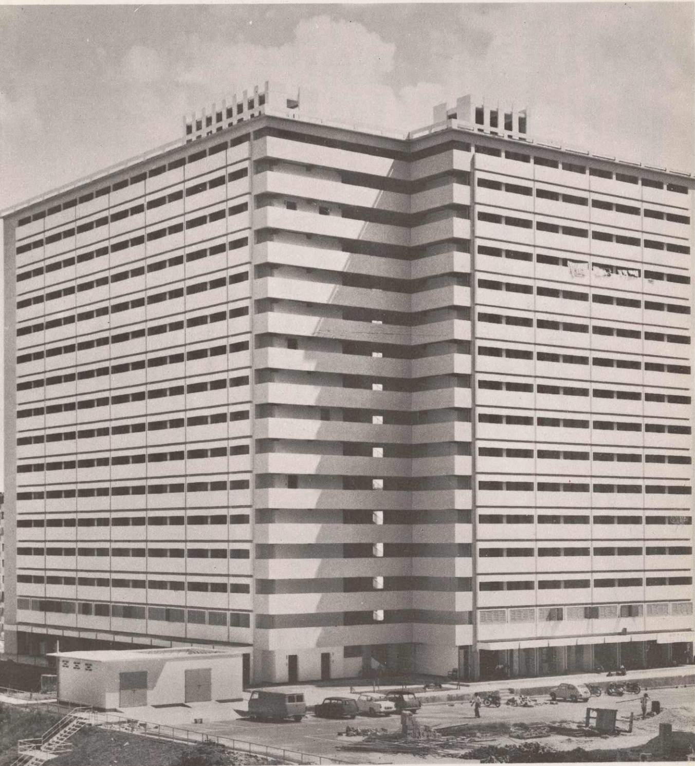
A newly-completed "L"-shaped block of 16-storeys containing 3-room improved flats in Neighbourhood 6, Queenstown.
