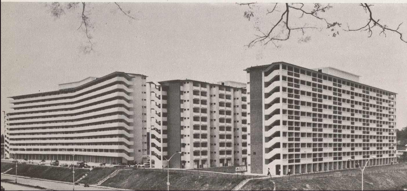
3 blocks of 10-storey 3 room improved flats in N4, Toa Payoh, which have been sold under the "Home Ownership for the People" Scheme.
