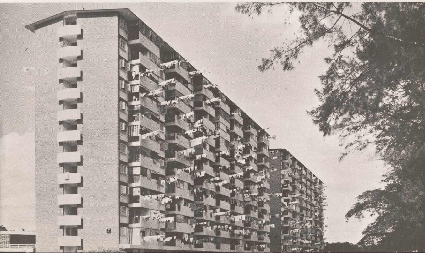
Two 12-storey blocks of 1-room improved flats with ground floor shops in Upper Aljunied Estate.
