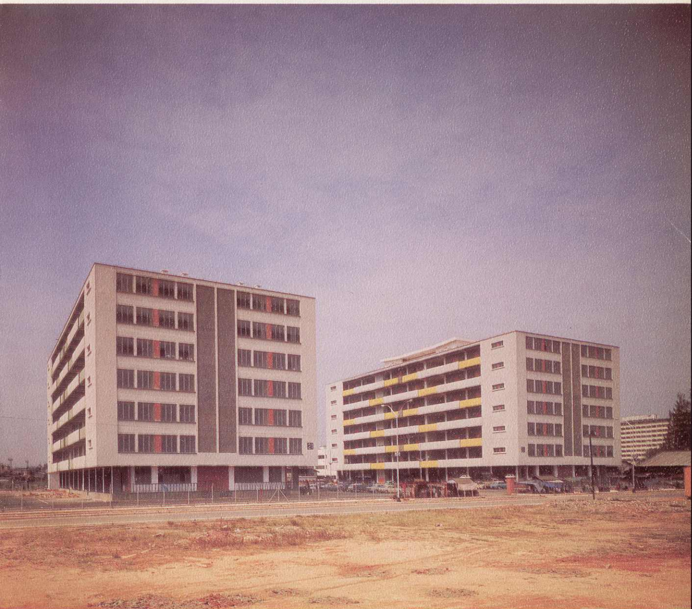
Close-up of the two blocks of 7-storey flatted factories at Kallang Basin Estate.
