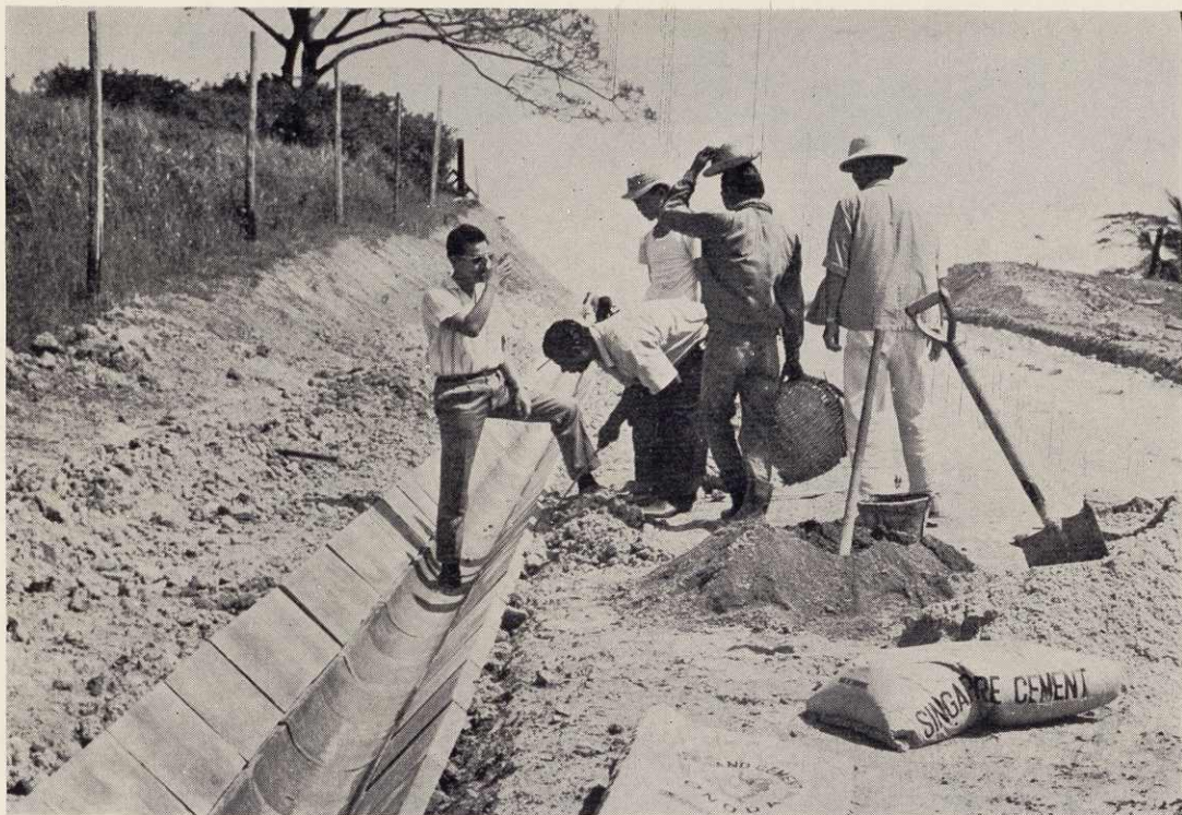
(7) Drains being laid in a Resettlement Area.
