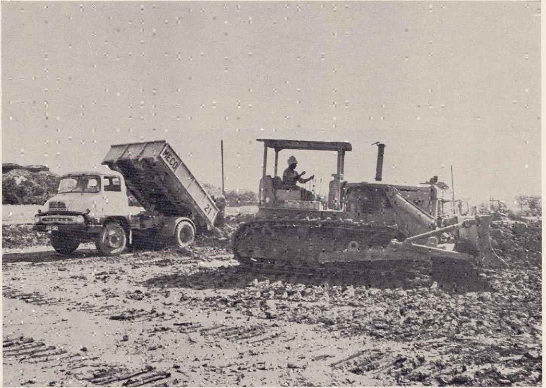
Excess earth from Toa Payoh being unloaded at Kallang Basin.
