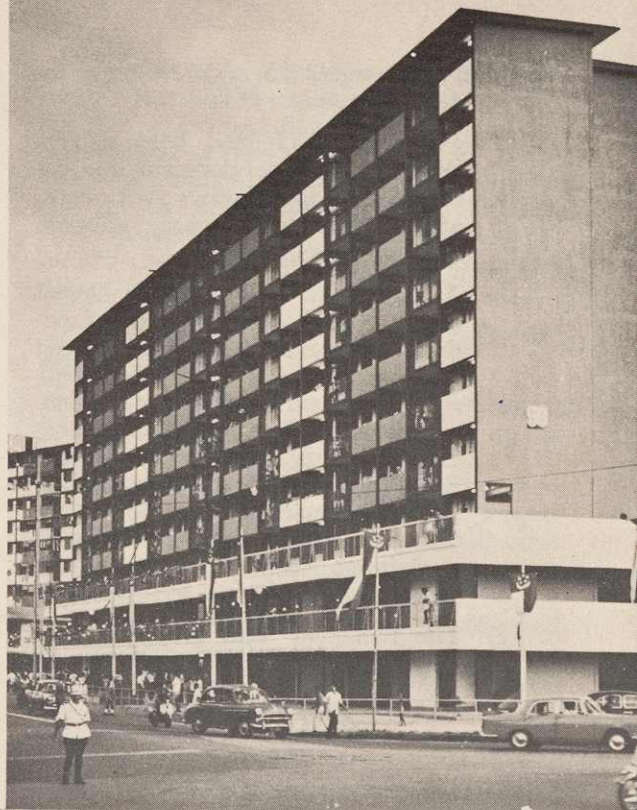
Hawkers Centre at Bukit Ho Swee Estate. Cooked food stalls on ground floor and dry goods on first floor.
