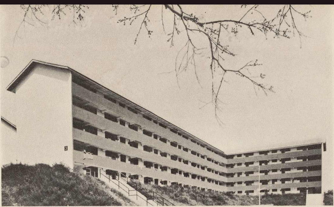
5-storey 2 & 3 Room Flats at Upper Changi Estate for the Resettlement of the people affected by the East Coast Reclamation.
