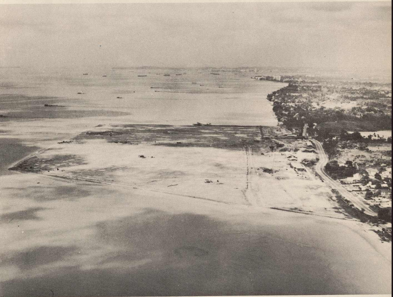
Aerial View of the East Coast Reclamation.
