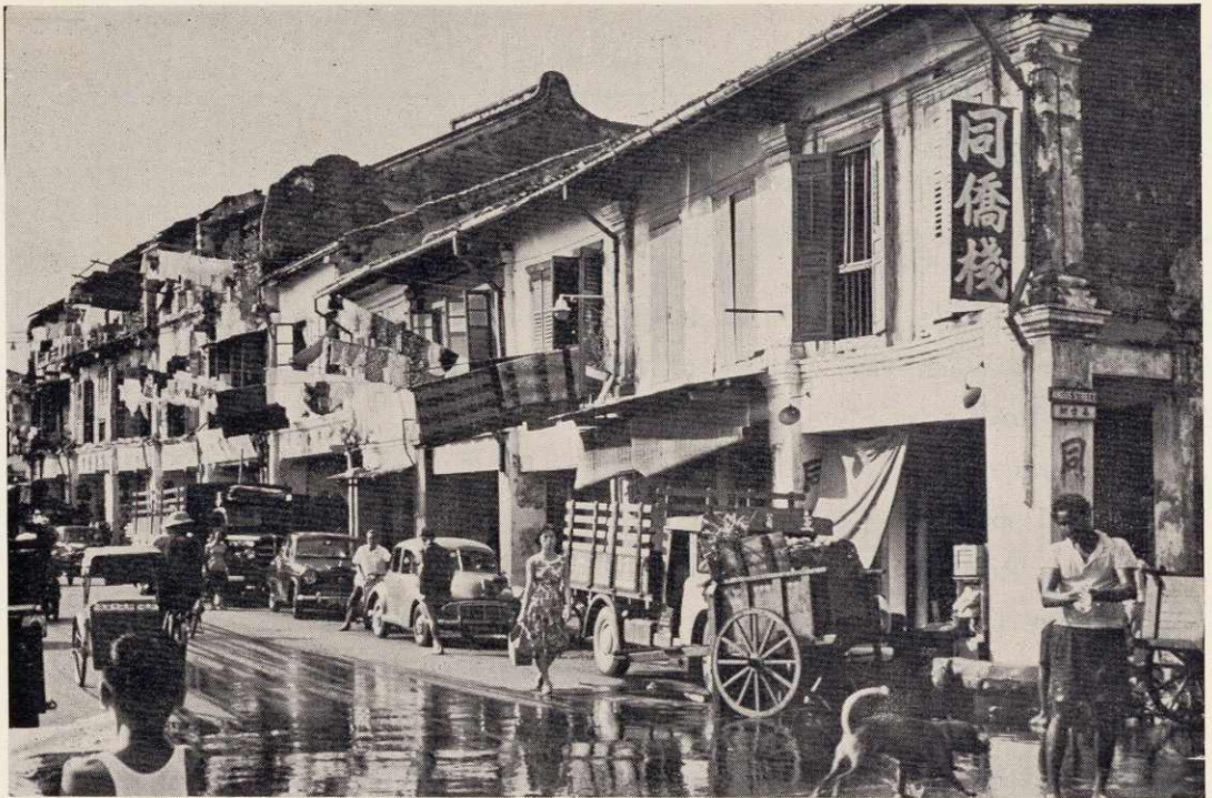
(1) Obsolete properties in the urban centre scheduled for clearance. Some 9,500 families have to be cleared from such properties in Precincts N1 & S1.
