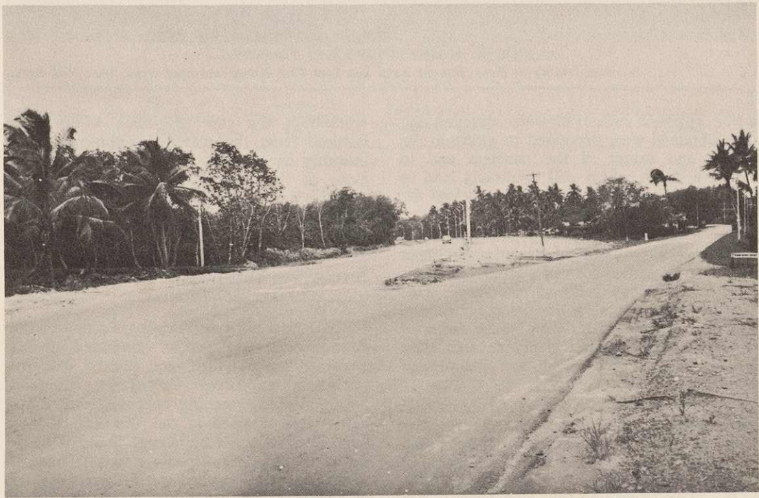
View of widened road after clearance.
