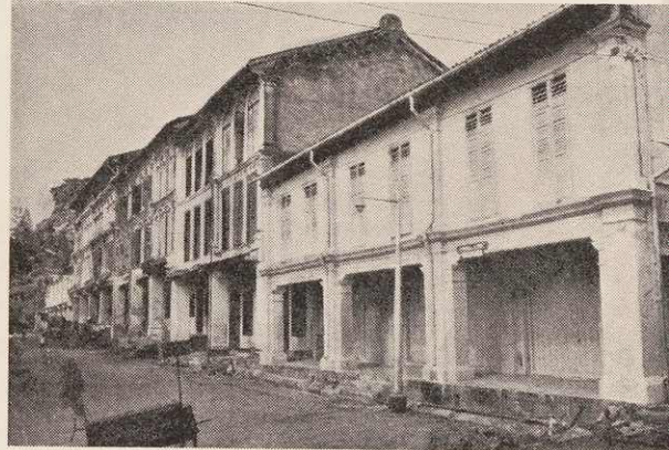
Old shophouses in Precinct S1 scheduled for demolition.
