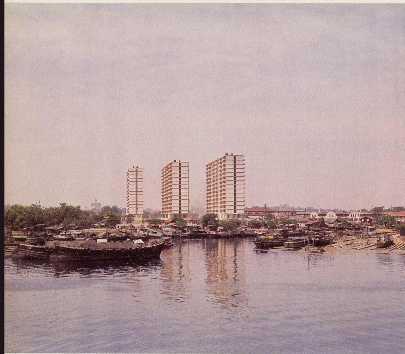
Contract 1A at Northern Precinct No. 1 Palembang Road Redevelopment under the Urban Renewal Programme.
