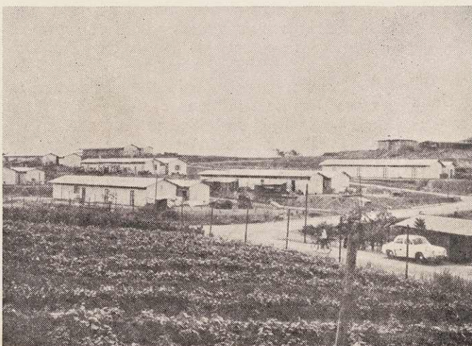
Basic Terrace Houses in Resettlement Area 53A for Malay Families affected by Clearance in Jurong.
