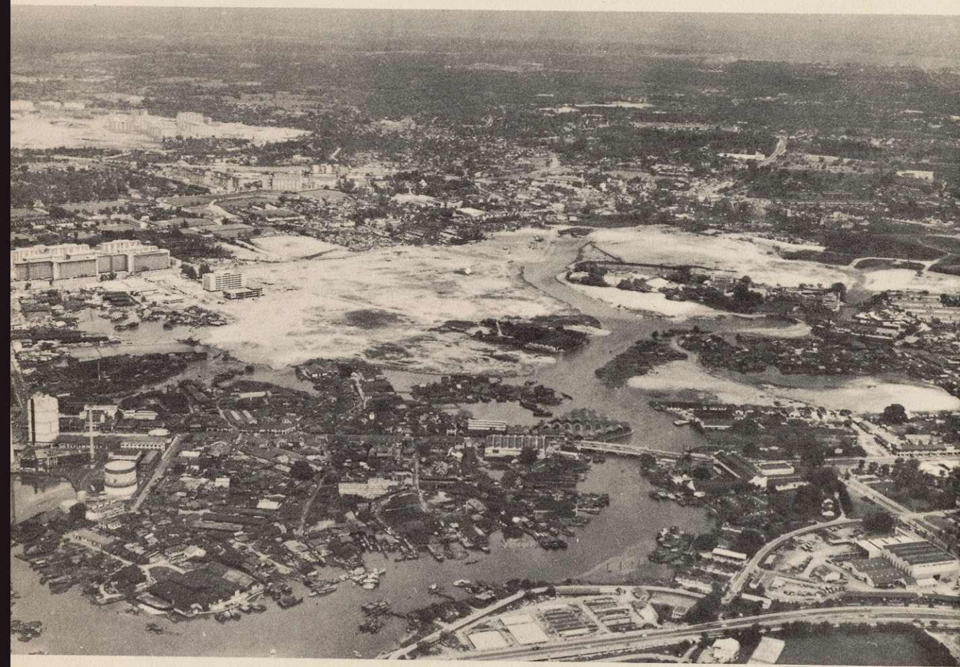
Aerial View of Kallang Basin Reclamation.
