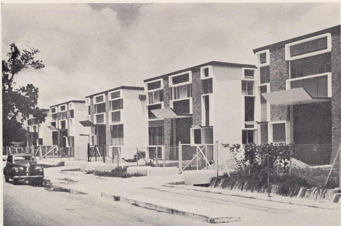
Kampong Ampat Industrial Estate: Front view of 5 detached 2-storey Standard Factory buildings.
