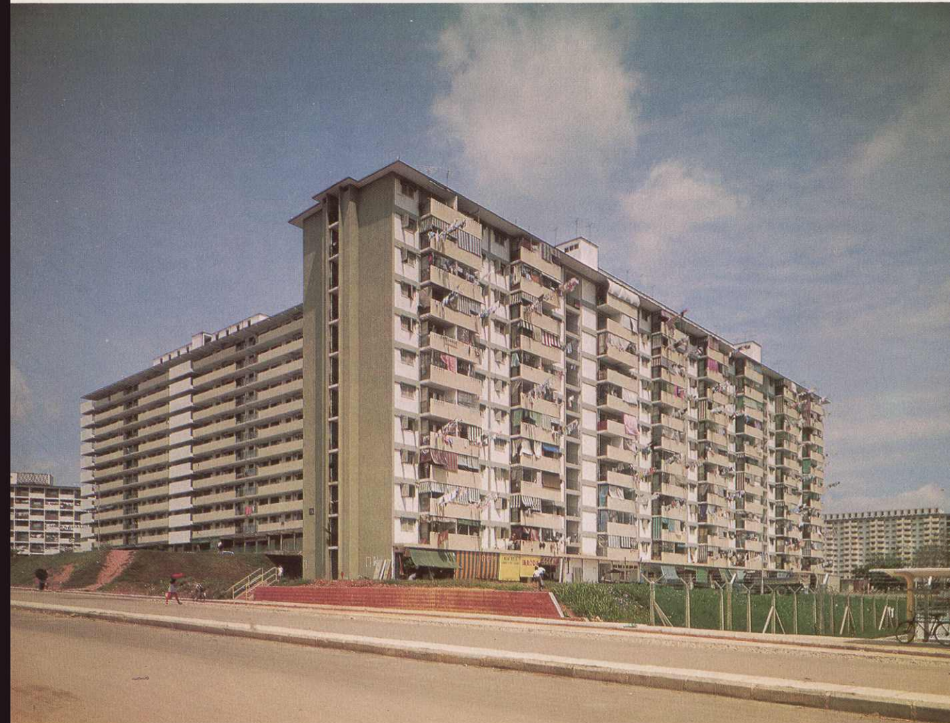
2 blocks of 12-storey flats with ground floor shops in Kampong Tiong Bahru.
