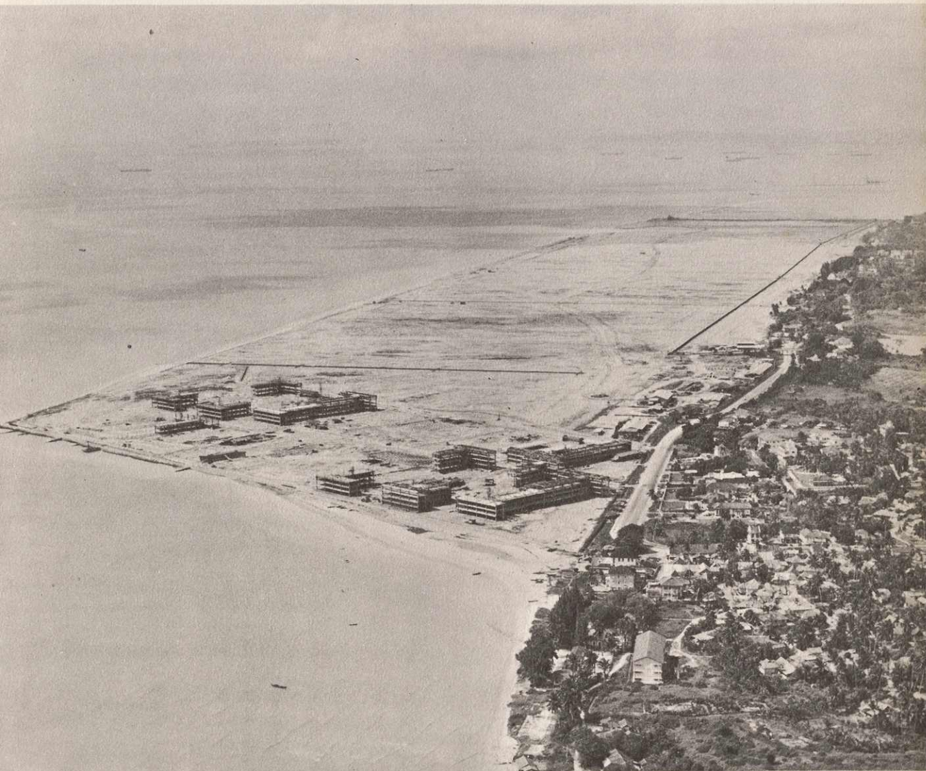
Aerial view of the East Coast Reclamation where more than 400 acres of land have been reclaimed by the end of 1967.
