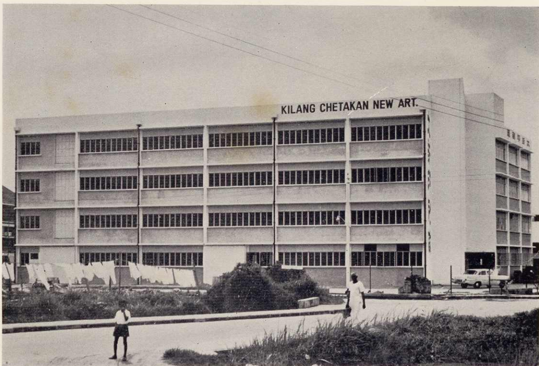
Kampong Ampat Industrial Estate: Colour Printing Factory.
