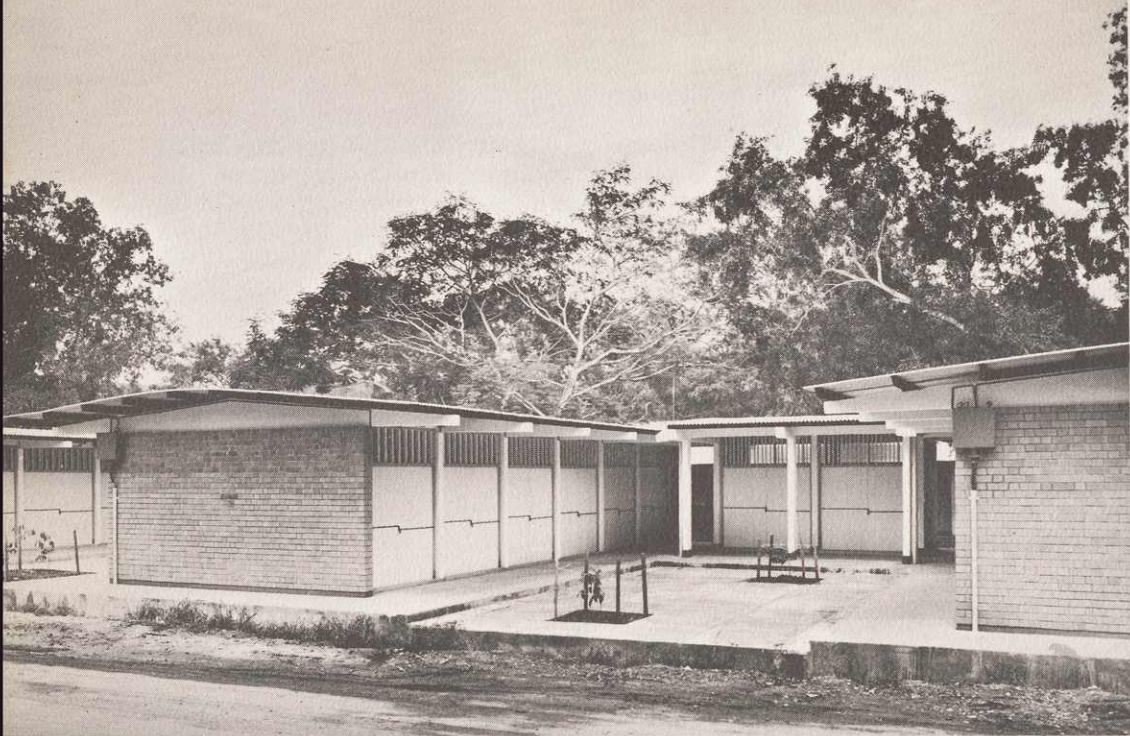
View of newly completed Hawkers' and food stalls in a Board estate.
