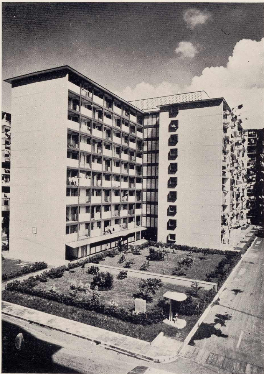
One of the blocks of multi-storey flats at Bukit Ho Swee with the Area Office on the ground floor.
