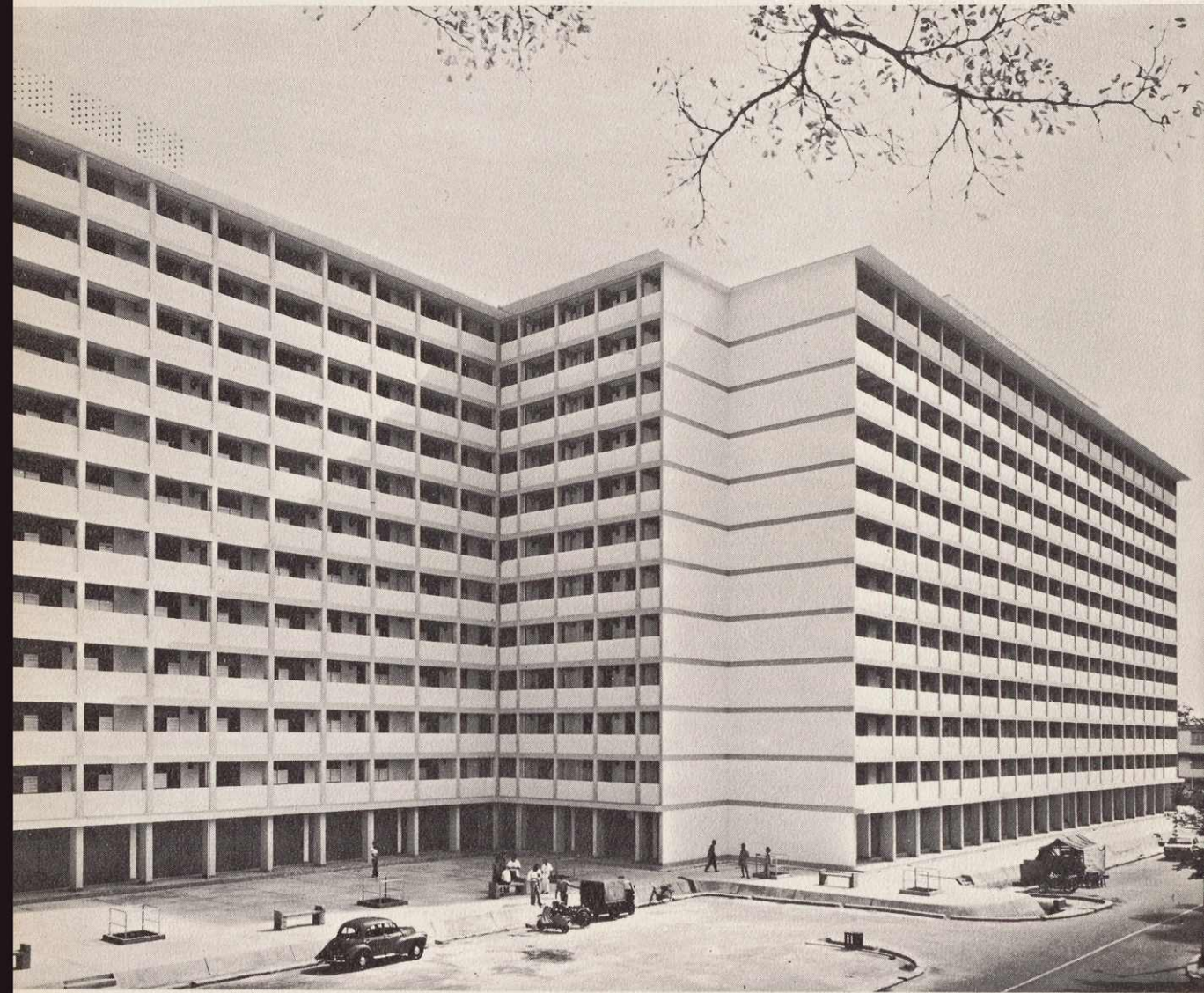
12-storey flats built for workers in Kallang Industrial Estate.
