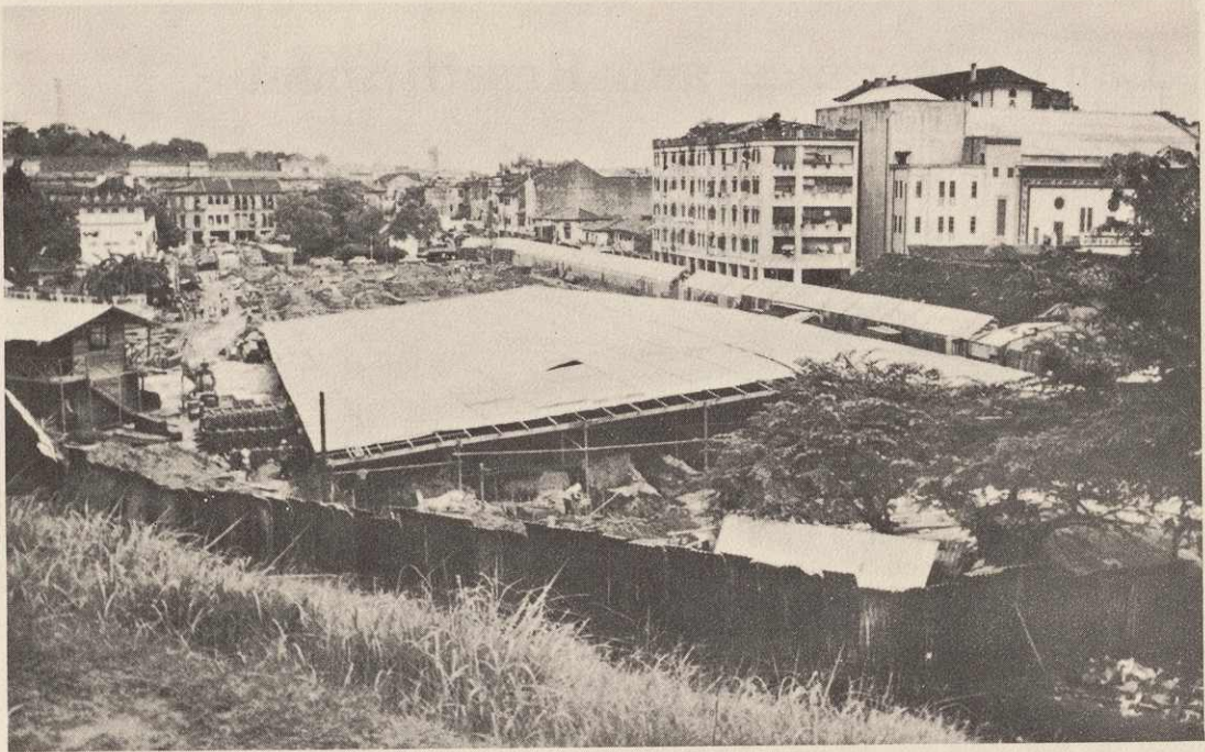
Building Construction in Progress for Park Road Redevelopment (Contract II).
