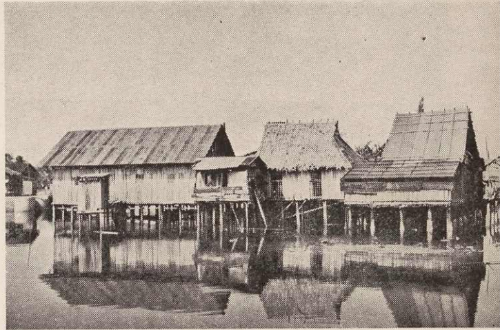
Examples of squatter huts at Kallang Basin which have to be cleared prior to reclamation.
