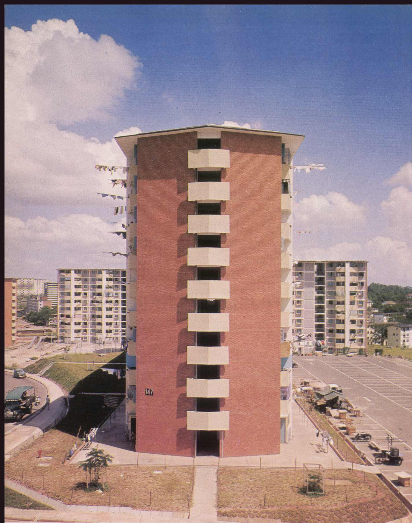
Side elevation of a 10-storey block of 1-room improved flats at Neighbourhood 6, Queenstown showing the Central Common Corridor.
