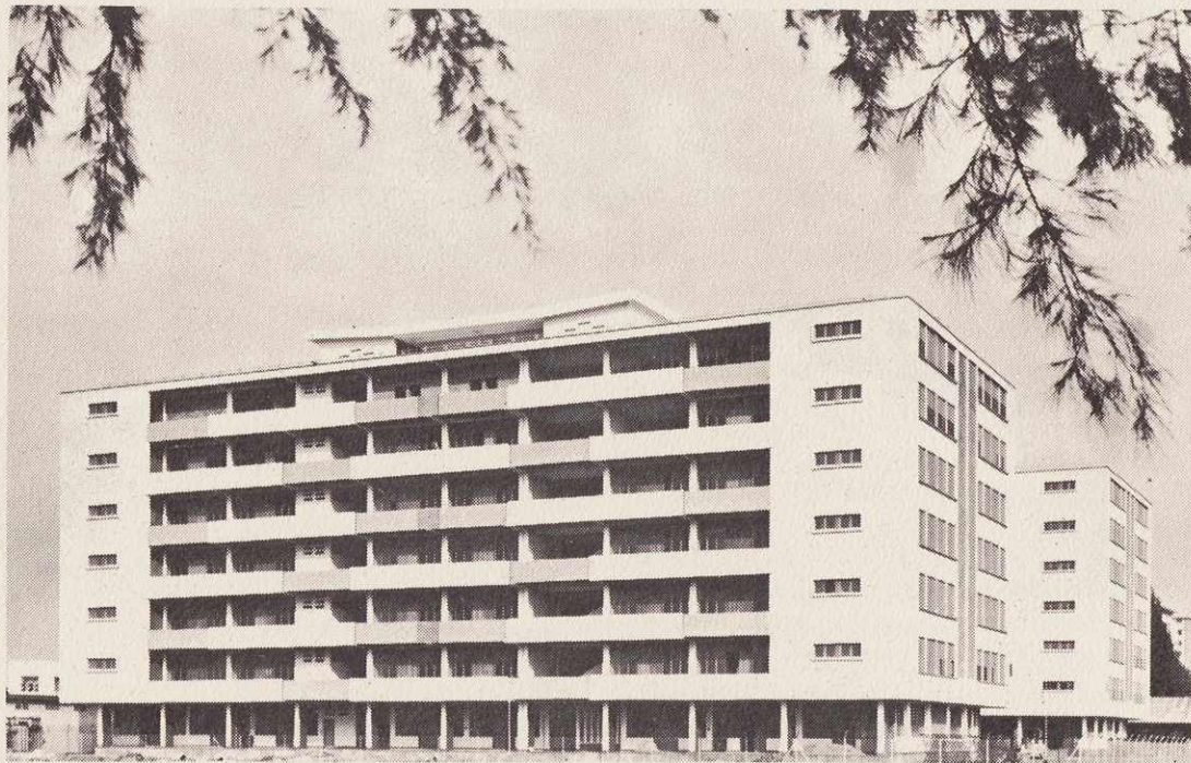
A closer look at the flatted factories at Kallang Basin Estate.
