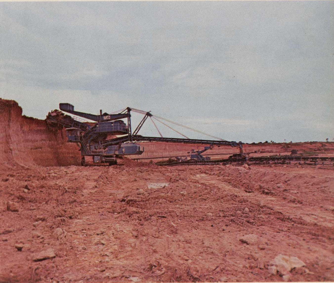
Giant bucket wheel excavators cutting the earth at Bedok Plain.
