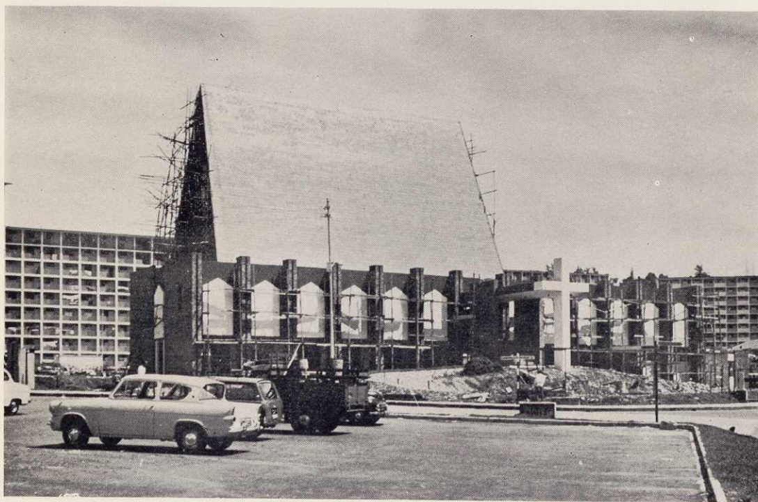
Church building under construction in Queenstown N. III.
