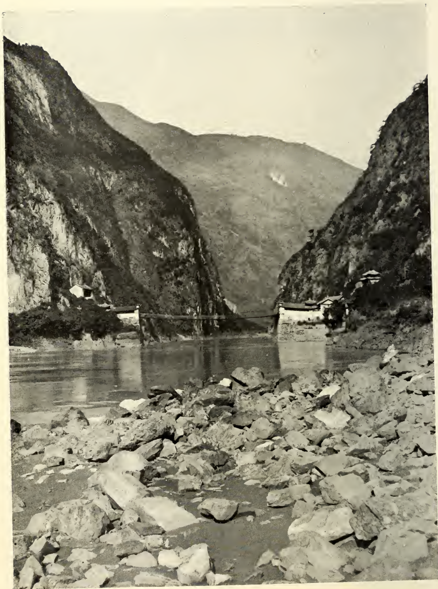
FIG. 17.—CHINESE CHAIN SUSPENSION-BRIDGE ON THE MEKONG. SPAN 75 YARDS. LOW WATER (SPRING) LEVEL.
