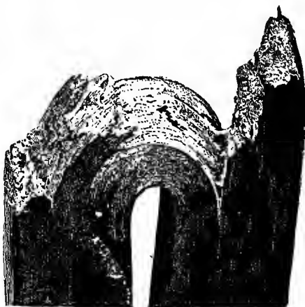
FIG. 115.—FRACTURE AT ORDINARY TEMPERATURE.
