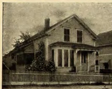
A No. 015 IDEAL Boiler and 175 ft. of 38-in. AMERICAN Radiators, costing the owner $118, were used to Steam heat this cottage.
