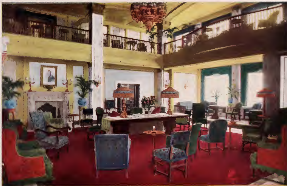
Grand Lounge Showing Sun Parlor and Mezzanine Floor
