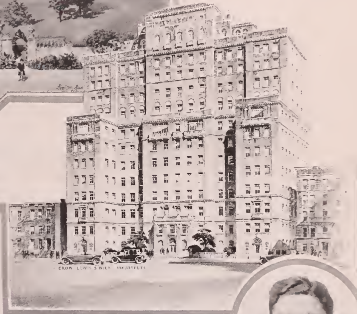
THE NEW FRENCH HOSPITAL NEW YORK CITY (Under Construction)
