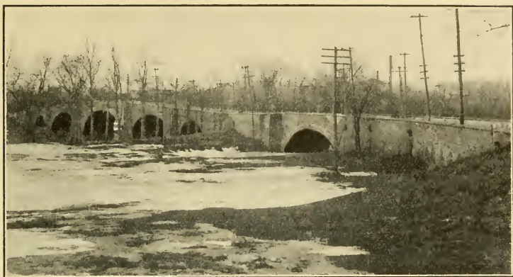
PERKIOMEN BRIDGE AT COLLEGEVILLE.
