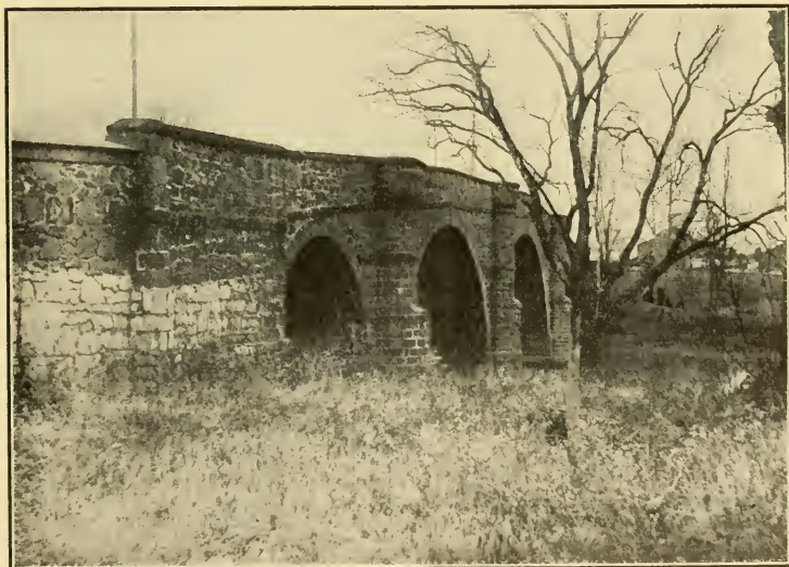
DETAIL OF THE SAME BRIDGE.
