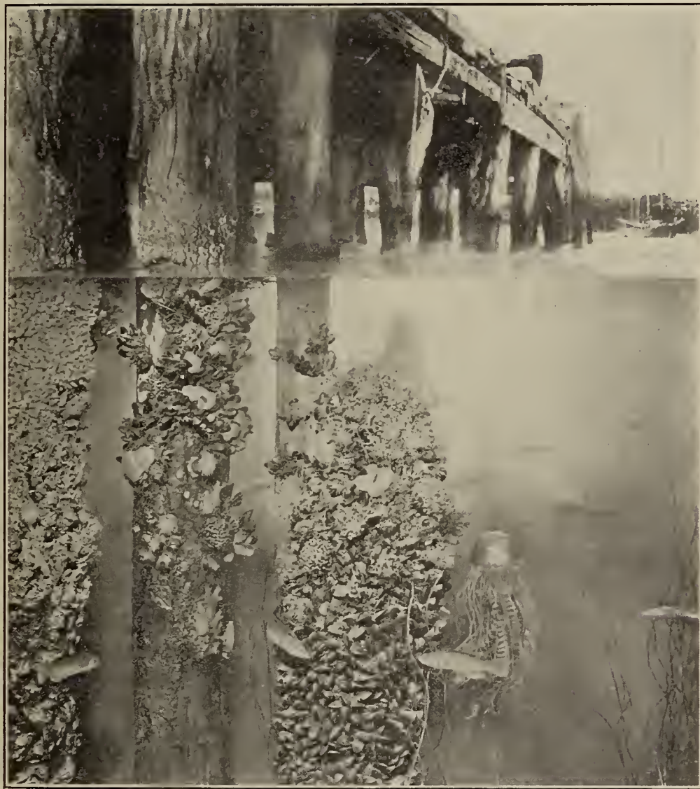
THE VINEYARD HAVEN WHARF PILE GROUP.
