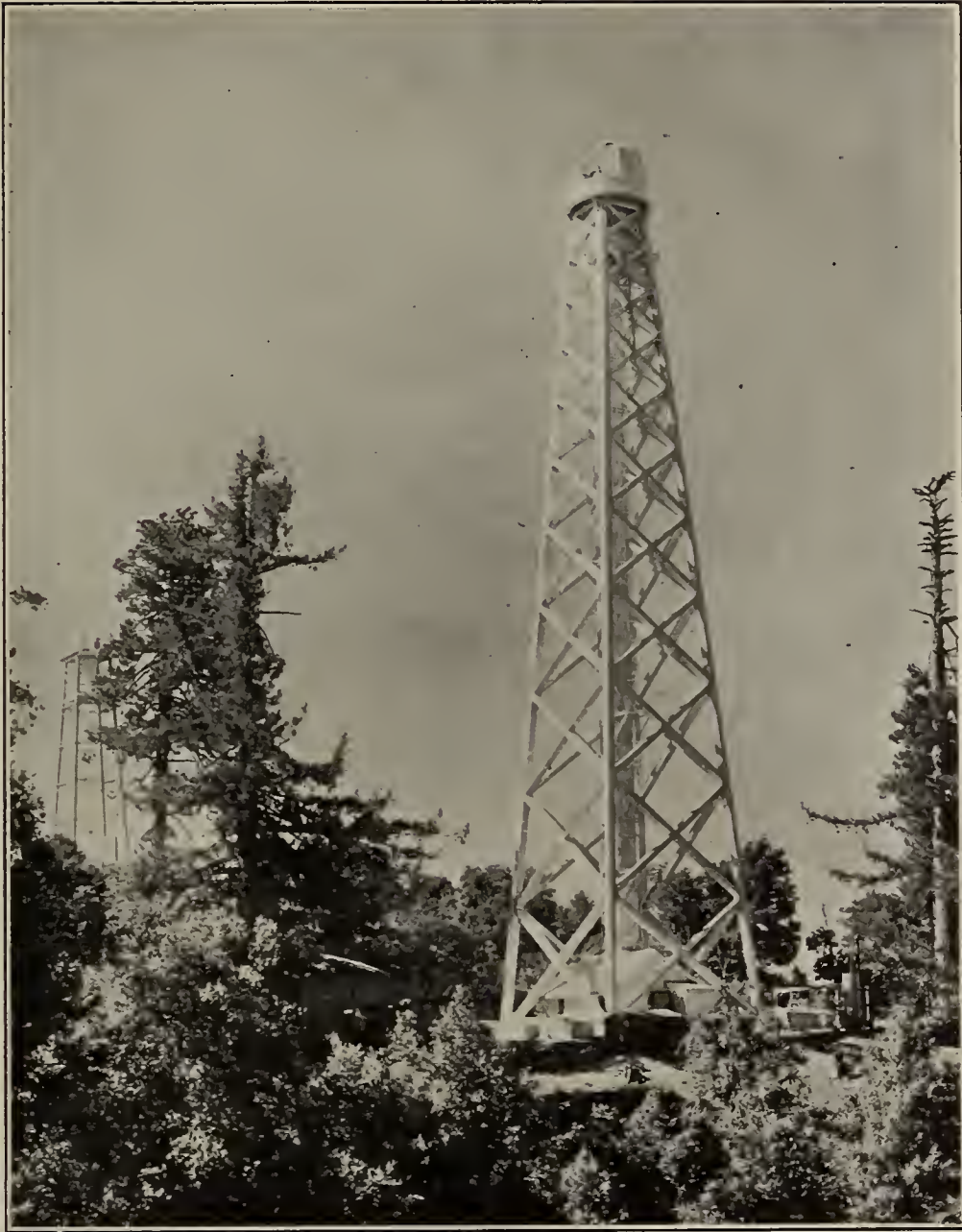
FIG. 13. 150-FOOT TOWER TELESCOPE.
