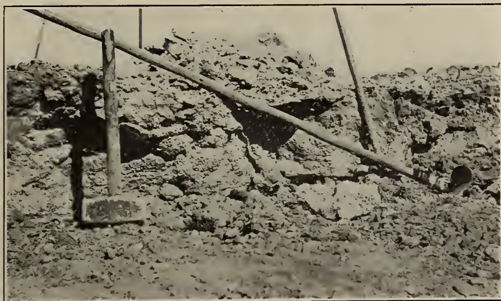
In a cutting which shows the layer of caliche with almost no overlying material. The tools shown are the only ones needed in mining caliche.
