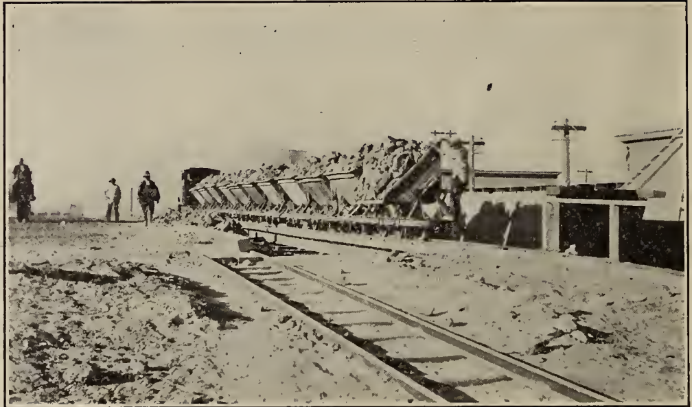
Dumping the caliche into the hoppers of the crushing machinery. Capacity of each car is about three tons.
