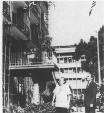
Administrative officers Mike Fink and Larry Alsbaugh check repairs on consulate building.
